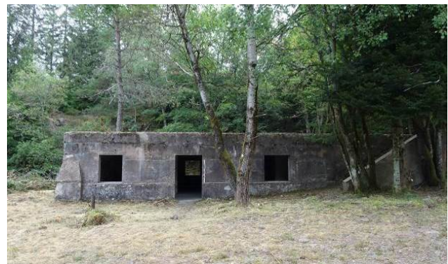
Figure 5: View of the southwest façade of the forge.
