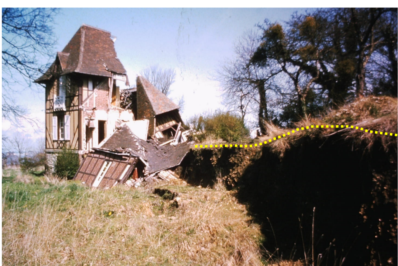
Fig. 2 - Destroyed building by the acceleration of January 1982 (Maquaire, 1985)
