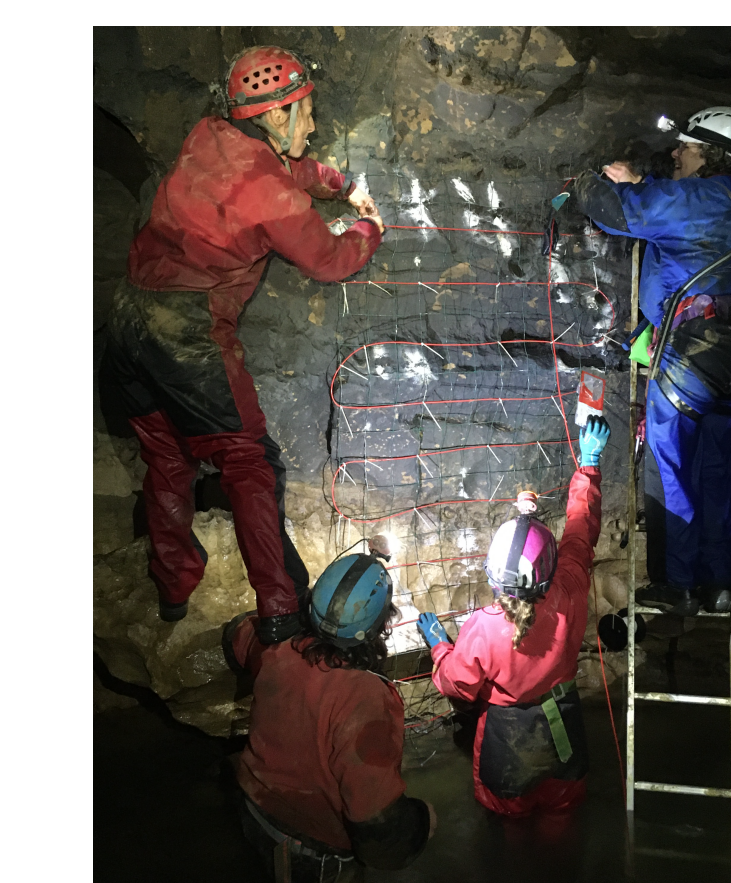
Fig. 9 : Installation of the optic fiber in a vertical plane for water level detection inside the cavity.
