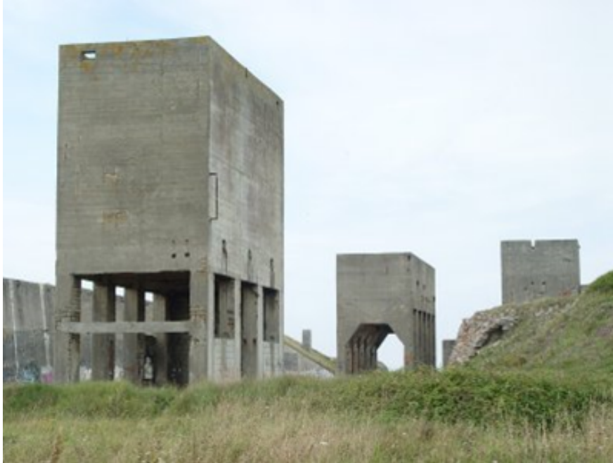
Figure 1.6. Remains of the pebble crushing plant of Tréguennec, Audierne Bay, France (source: C. Meur-Ferec, 1989). For a color version of this figure, see www.iste.co.uk/rebotier/risks.zip
