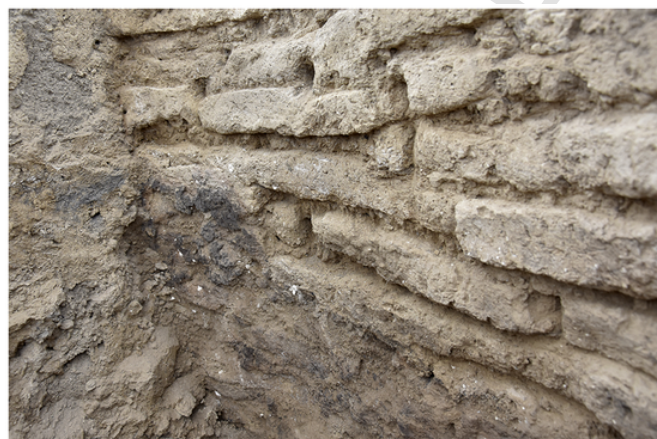
Fig. 17. Detail of the burnt coating and flat mud-bricks of STR 21, square G8, view from the north-west (Mission Boyuk Kesik, MEAE).
