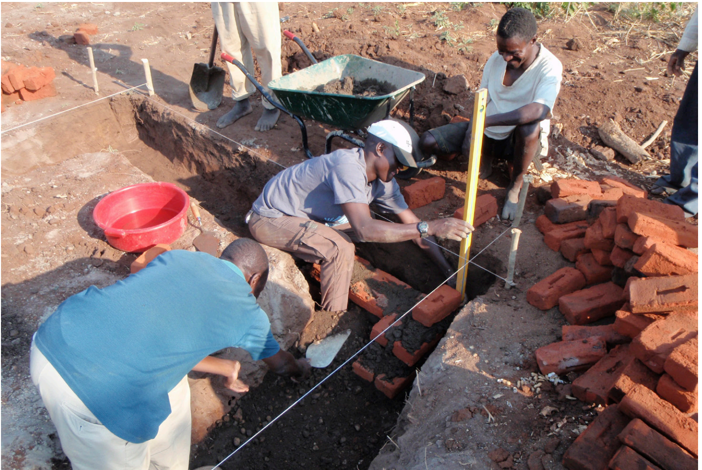
Construction of a foundation. CC- Gregory S.
