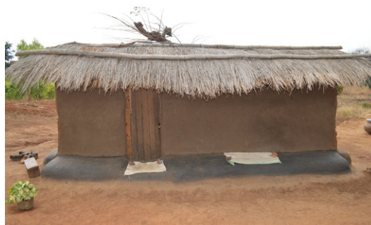
House built with on a raised platform with wattle and daub walls and thatched gable roof. Mkalawa, Rumphi.
