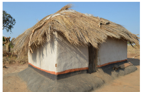
Low-rise houses with round and compact forms and symmetric and scarce openings and light roofs are good to resist seismic forces. Round house in Kachipeso, Dowa (top). Square house in Muwanga, Chitipa (bottom). © Jon Twingi
