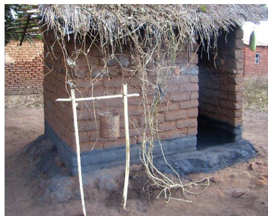
Hand-washing facility outside a pit latrine.
