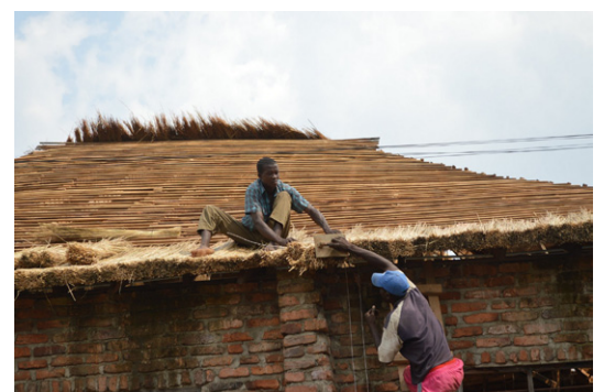
Thatch roof under construction in Sifukwe, Karonga. © Jon Twingi
