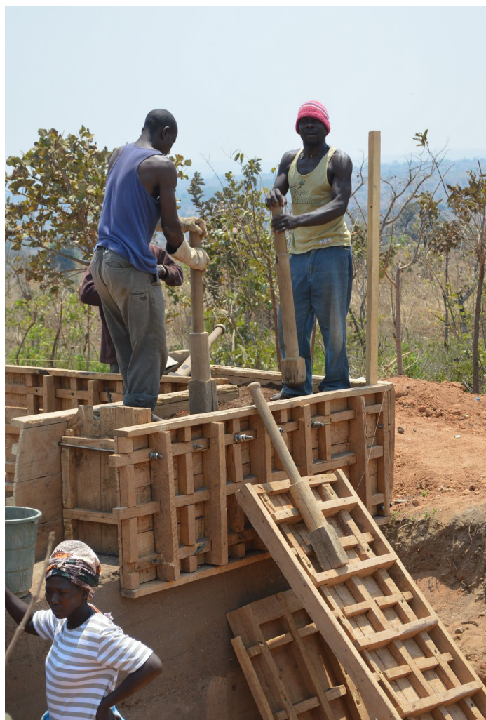
In some areas, there is a need to help one another build their home. Construction of a rammed earth house in Nisanje, Lilongwe. © Jon Twingi
