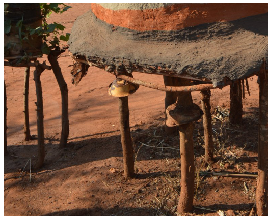
This granary in M'buka (Kasungu District) has metallic barriers in order to impeach rats and other small animals to reach the food. © Jon Twingi
