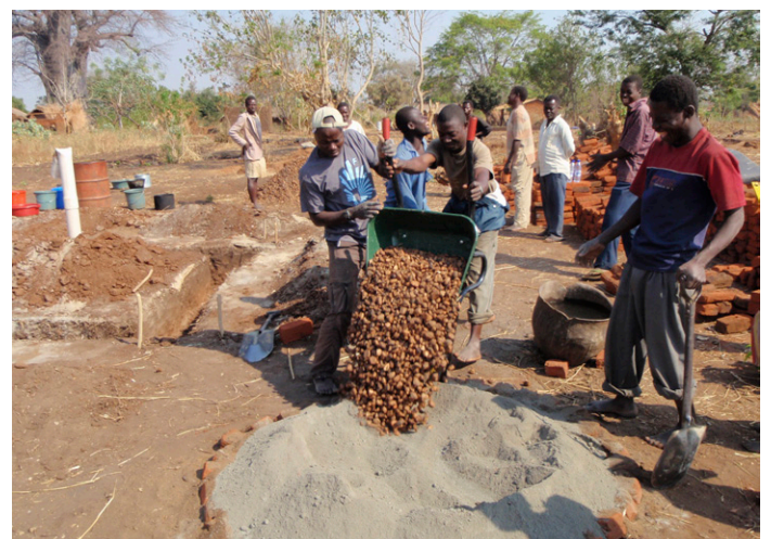
Stage of construction of foundations of a house.
