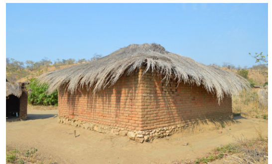
Stone foundation and plinth (Chimwendo, Karonga) protecting the walls from humidity and floods. © Jon Twingi.
