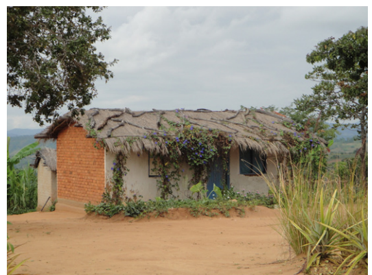
House with burnt brick walls, thatched gable roof protected from the winds with timber elements on it and a plaster to protect the main façade from the driven rain. CC- May N.
