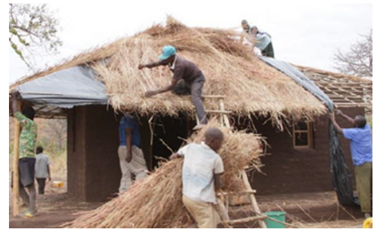
Image of the construction process. © Jamie Richardson (CRS)
