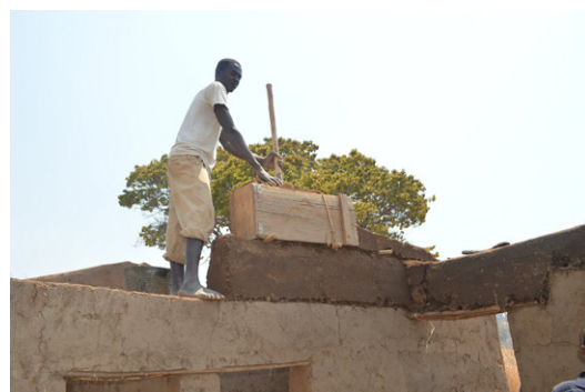
Rammed earth house under construction in Chimombo, Ntchisi. © Jon Twingi.
