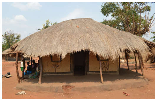
Verandas and large roof overhangs between the interior earth wall and the exterior avoid the risk that changes in humidity associated with rain will swell the soil under the walls. House in Simwaka, Nkhotakota. © Jon Twingi
