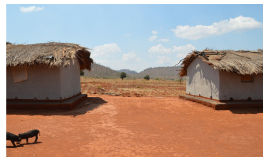
Distance between buildings is a good strategy to fight against the spread of fires. Most constructions in rural family homesteads are placed separately ones from the others. Homestead in Gausi, Nzimba. © Jon Twingi
