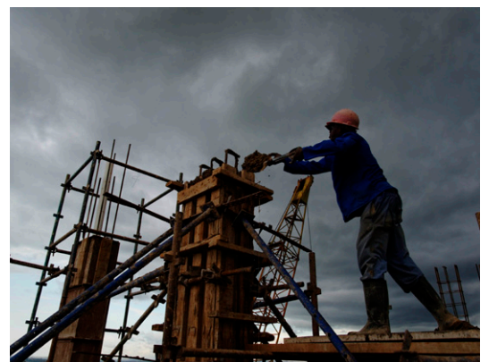
Reinforced concrete construction in Lilongwe. CC- ILO
