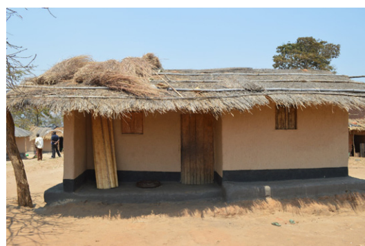
Longitudinal bamboo or timber pieces are sometimes joined to the roof's structure for better resistance to wind. House in Nyemba, Kasungu. © Jon Twingi
