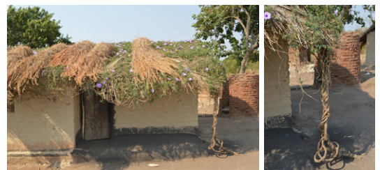
In some villages, the roof is used as a support for climbing plants. The risk of wrenching as well as partial or total uplift is reduced as the plants fasten together the roof components and attach the roof to the ground through the roots. House in Nsangu, Salima. © Jon Twingi
