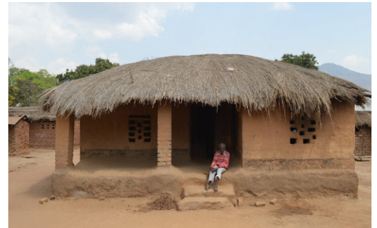
Houses constructed using adobe bricks, render and earth mortar like this one (Chisoka, Rumphi District) responded well to the important floods in 2015 (CRS, 2020) as the design developed over centuries provides protection from the elements. Other than some minor repairs, some of these houses were in good condition and allowed the families to return to their homes once the floods had subsided. © Jon Twingi
