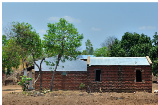
Corrugated galvanised steel or iron sheets are the most common metal roofing system in Malawi. Houses in Makala. CC- Hansueli Krapf
