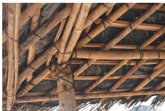
Plastic sheet membrane in a roof in Chipile, Mangochi. © Jon Twingi
