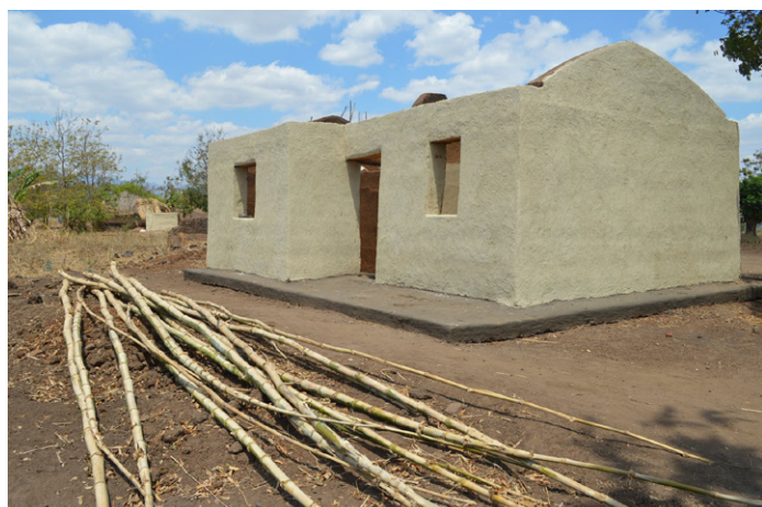
Rammed earth house under construction. © Jon Twingi
