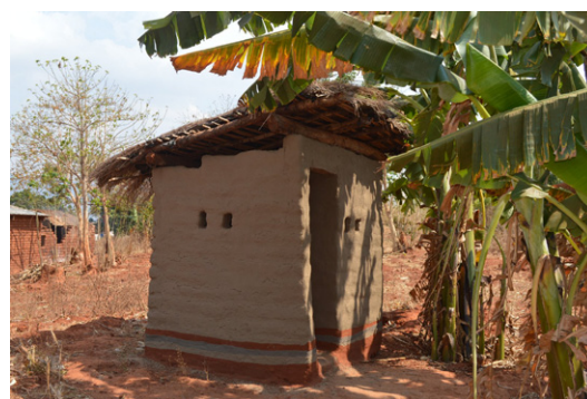
Latrine in Chome, Rumphu. © Jon Twingi
