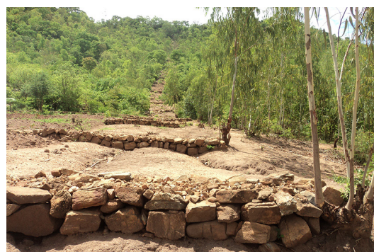
Stone bunds are a solution to reduce the speed of surface water and promote the penetration of water into the soil, thus avoiding erosion. Example of stone bunds built by Khole community in Machinga district. © PCI
