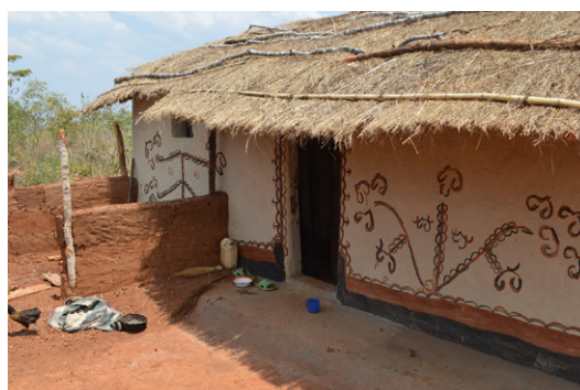
Extensions are very common. More often, new constructions are built in the same plot completely separated from the existing ones. This house is in Mwamkenja, Chitipa. © Jon Twingi
