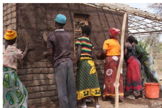
Images of the construction process.
