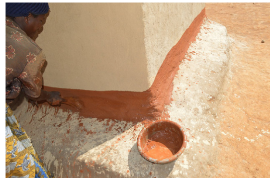
Woman applying a red earth based painting in Chisi, Nzimba. © Jon Twingi.
