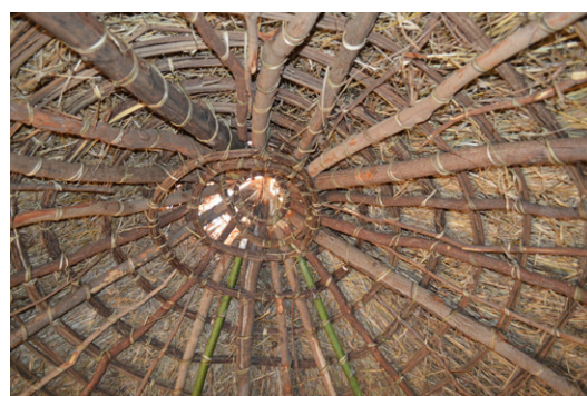
Roofing frameworks are often built with timber poles (usually blue gum), but also with bamboo. Conical roof in Bushiri, Salima. © Jon Twingi.
