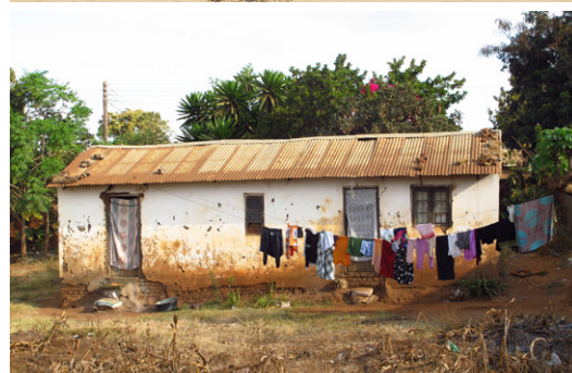
These two houses would be semi-permanent according to different authors as they are built with a mix of materials. The one on top has burnt bricks and thatched roof (Kachopatsonga, Nkhata Bay- © Jon Twingi). The other one has adobe brick walls and metallic roof (Lilongwe- © Urbanopolista)
