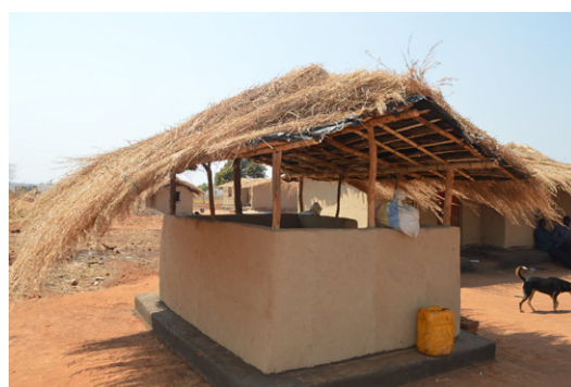
Kitchen with the upper parts of the walls open for improved ventilation. Nkhombe, Kasungu. © Jon Twingi
