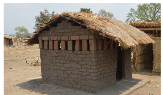
Small openings in the masonry walls allow adequate ventilation in the interior of the buildings, particularly in kitchens. Kitchen in Kalinyka, Ntcheu. © Jon Twingi
