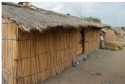
House built with timber or bamboo framework, wattle and daub walls, and thatched roof (thatch).
