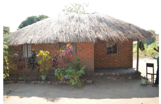
House built on a raised stone and earth platform with burnt brick walls and thatched hip roof. Sifukwe, Karonga. © Jon Twingi
