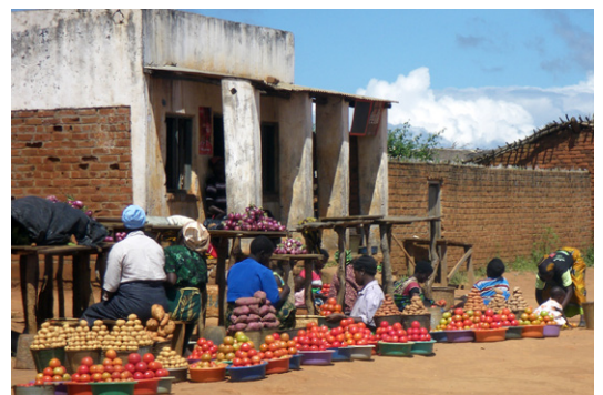
The roof of the veranda ( khonde ) is structurally independent from the main roof of the building in order to avoid damage to the main building roof during strong windstorms. Construction in Karonga. © Sonia Molina
