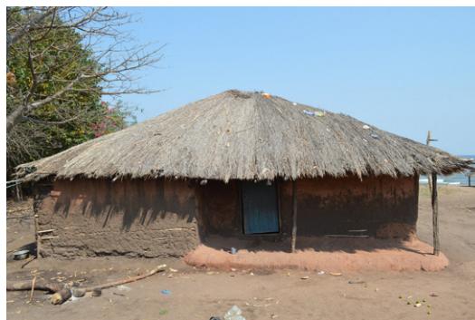
House with veranda built on a raised platform with wattle and daub walls and thatched hip roof. Mkwamwiyo, Karonga.
