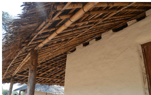
House in Dzipusile, Ntcheu. This house has a contact surface between the wall and the roof structure which is minimised using only some bricks to sustain the framework. This permits ventilation, but also allows for a better visual detection of termites paths and thus a better control of their attacks. © Jon Twingi
