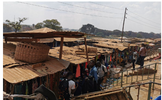
The use of CGI sheets without false ceilings and without ventilation in the gables causes thermal and acoustic discomfort. Market in Lilongwe. © Roderick Vd.
