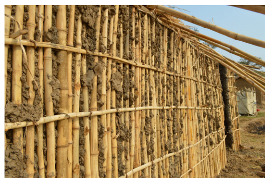
Wattle and daub house under construction in Chipita, Karonga. Bamboo framework and earth mortar. © Jon Twingi.
