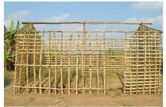
Light structures are good solutions in the event of an earthquake as even if they fall they are less likely to cause damages. Structure of a wattle and daub house in Mwaluwimba, Karonga. © Jon Twingi
