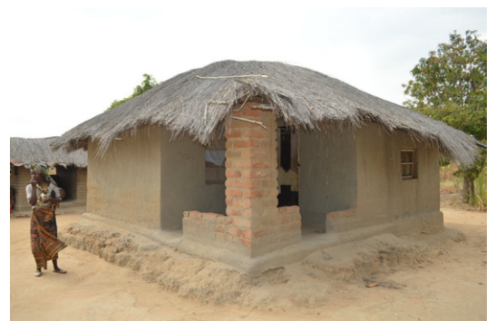
House with veranda built on a raised platform with burnt brick walls and hipped roof covered with thatch. Mariata, Nkhata Bay. © Jon Twingi
