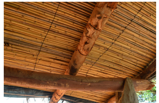
Reed is used as bottom layer in many roofs. Roof in Chome, Rumphi. © Jon Twingi.
