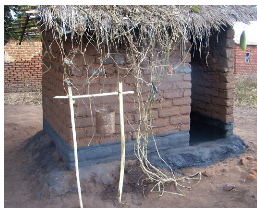
Hand-washing facility outside a pit latrine.
