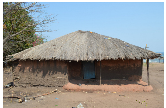
House with veranda built on a raised platform with wattle and daub walls and thatched hip roof. Mkwamwiyo, Karonga. © Jon Twingi
