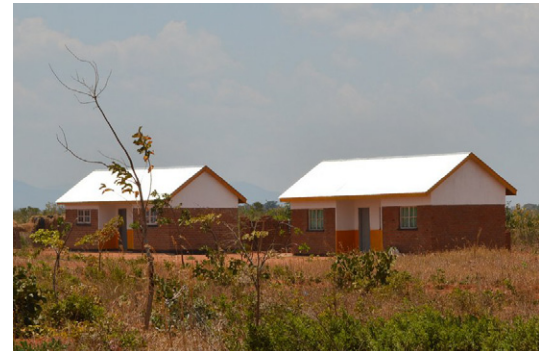
Houses with burnt brick walls, Reinforced Concrete beams and window sills, CGI sheets roof in Chisusu, Nzimba. © Jon Twingi
