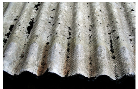
Corrugated asbestos cement roofing sheet. CC- Leo Reynolds
