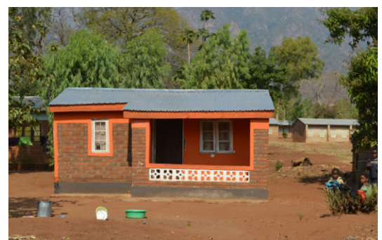
House with veranda built on a raised platform with burnt brick walls and gable roof covered with light metal sheets. Gawanani, Zomba. © Jon Twingi
