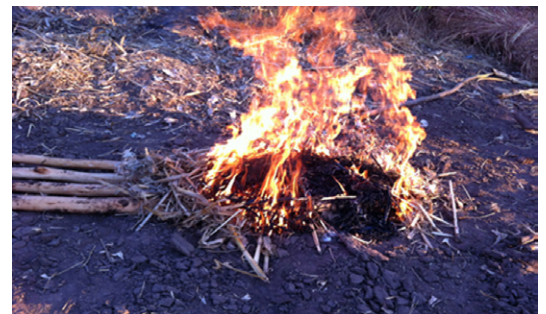
Timber poles are burnt to prevent termites' attacks before being inserted on the ground. Phalombe District. © CADECOM
