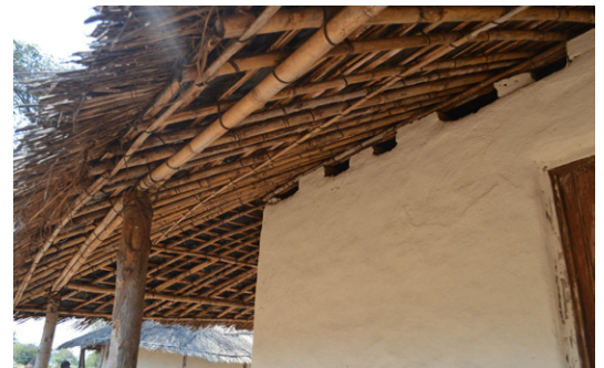
House in Dzipusile, Ntcheu. This house has a contact surface between the wall and the roof structure which is minimised using only some bricks to sustain the framework. This permits ventilation, but also allows for a better visual detection of termites paths and thus a better control of their attacks. © Jon Twingi
