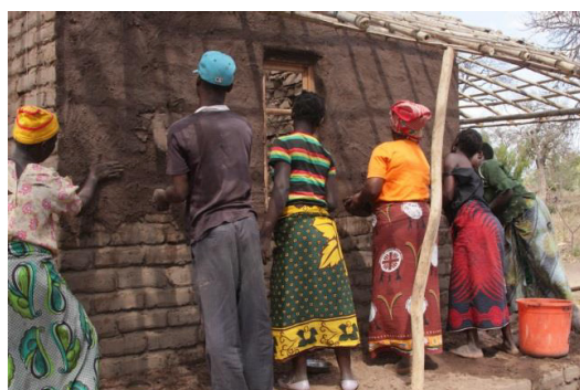
Images of the construction process.
