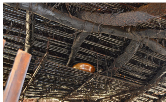
Raised platforms inside the houses are used to store food and seeds, preventing them to be damaged by floods. House in Chakhutupa, Chitipa. © Jon Twingi
