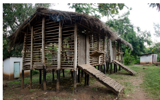
Raised constructions help protect small animals like goats or chicken from floods. These constructions are very common throughout the country. This is an example of raised goat pen at Naming'azi Farm Training Centre. CC- Carmichael C.
