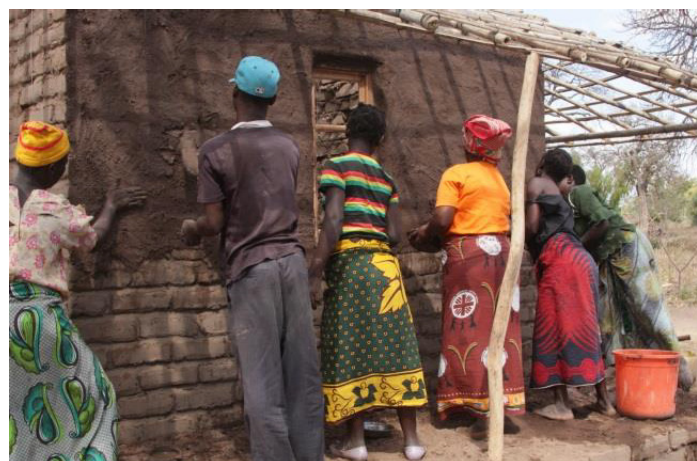
Rendering a house in a training by CRS. © CRS
