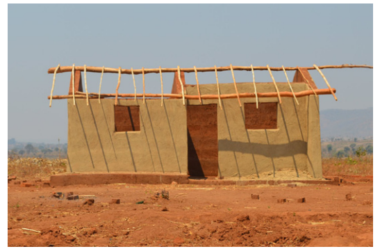
House under construction with rammed earth walls. Chimombo, Ttchisi. © Jon Twingi
