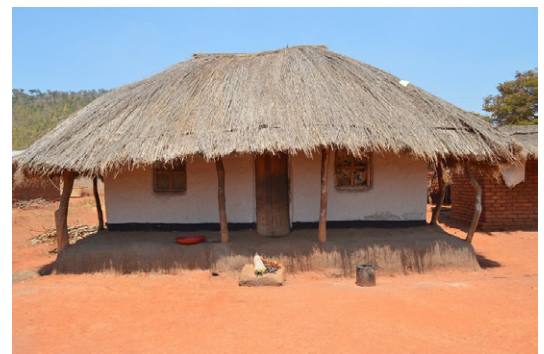
House built on a raised platform with a four sides veranda and a thatched hip roof and with its façades protected by a plastering and painted. Gama, Mchinji. © Jon Twingi .
