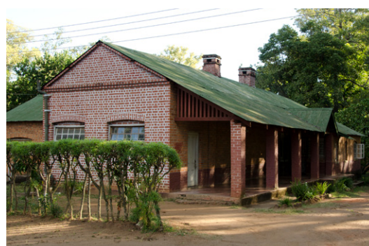
British colonialism also introduced in Malawi the use of fired red bricks, regular and paced windows and doors, concrete or burnt bricks lintels and roofs covered with corrugated iron sheets. Mission in building in Blantyre. CC- Carmichael C.
