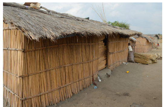
House built with timber or bamboo framework, wattle and daub walls, and thatched roof. Mkalawa, Rumphi. © Jon Twingi
