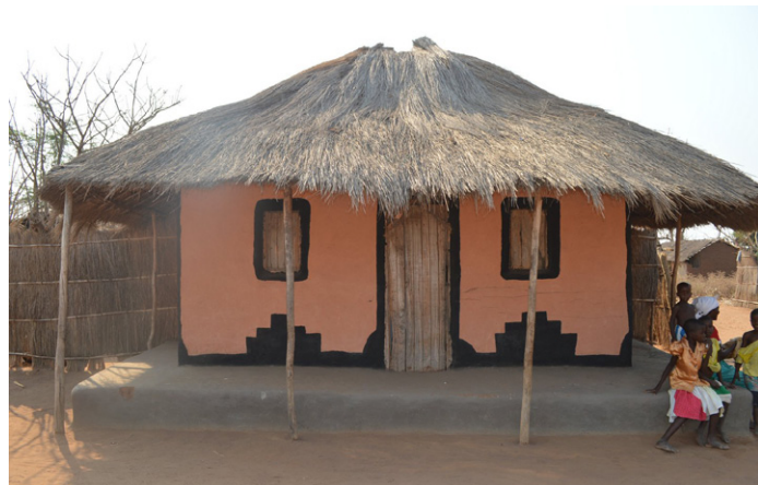
Decorated house with regular form and openings, thatched lightweight roof and four sides veranda (Malaza, Salima). © Jon Twingi
