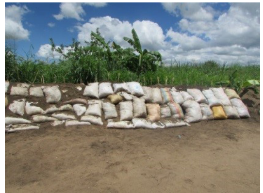
Riverbank stabilization with siltbags in Chilanga river in the zone of Kadzuwa village. © PCI
