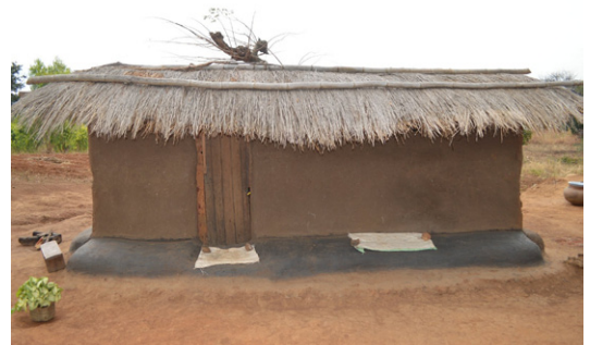
House built with on a raised platform with wattle and daub walls and thatched gable roof. Mkalawa, Rumphi. © Jon Twingi
