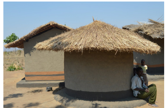
Round and rectangular plan constructions built on raised earth platforms in Juma, Dowa District. © Jon Twingi
