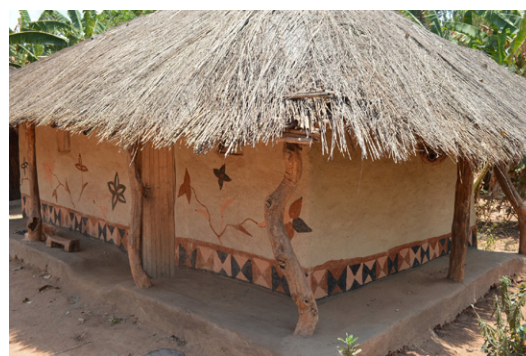
When a tree is cut down profit is taken of the whole tree. This is an image of the frugal use of resources as even twisted parts of good quality timber are used for the poles of the veranda. House in Kabomolo, Chitipa.
