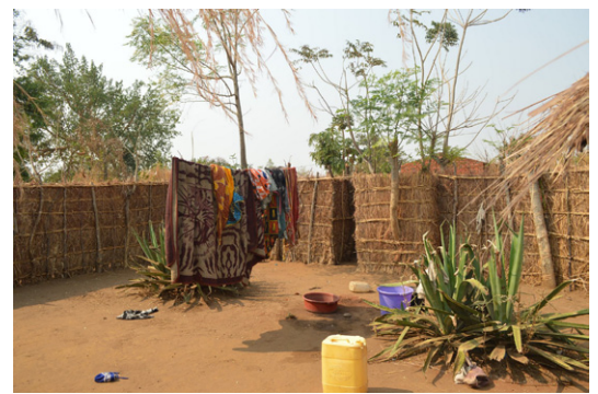
Bamboo, grass or reed fences are sometimes built to reduce the speed of wind and to delimitate plots. House in Lifidzi, Salima. © Jon Twingi
