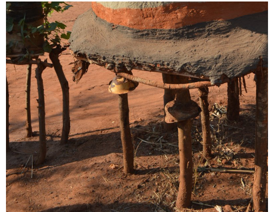
This granary in M'buka (Kasungu District) has metallic barriers in order to impeach rats and other small animals to reach the food. © Jon Twingi
