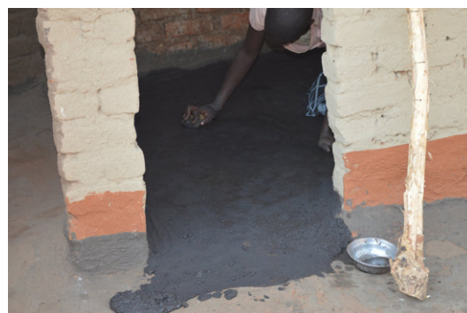
In some zones (e.g. Chaima, Dowa), used battery cells are cut and added to the mixture for earth floors. This can be a good practice regarding durability of plasters, but should be analysed also in regard to the health issues that it may cause. © Jon Twingi
