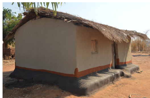
The earthen mounds are strengthened before the rainy season. The foundations are improved with an extra layer of mud. House in Chaima, Dowa District. © Jon Twingi
