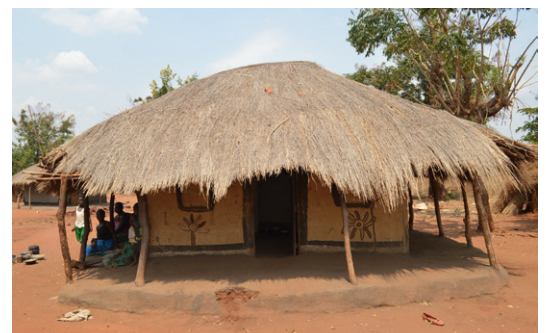
Verandas and large roof overhangs between the interior earth wall and the exterior avoid the risk that changes in humidity associated with rain will swell the soil under the walls. House in Simwaka, Nkhotakota. © Jon Twingi
