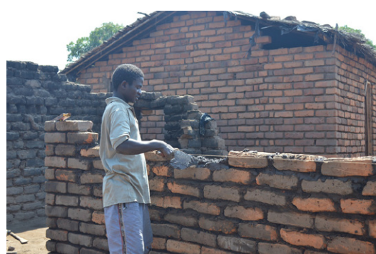
Burnt brick wall with cement mortar being built in Kambewa, Mulanje. © Jon Twingi.
