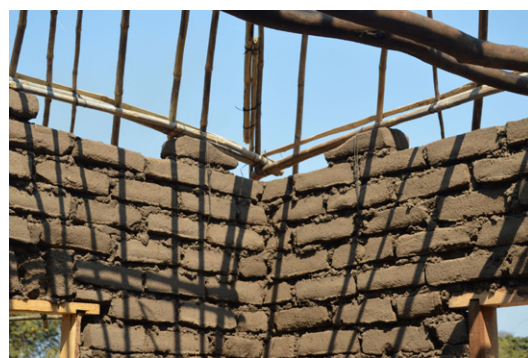
The roof structure is tied to the wall through several wrappings of galvanised metal wire, avoiding to wrap the metal wire in correspondence to vertical mortar joints. House under construction in Chakwela, Mangochi. © Jon Twingi
