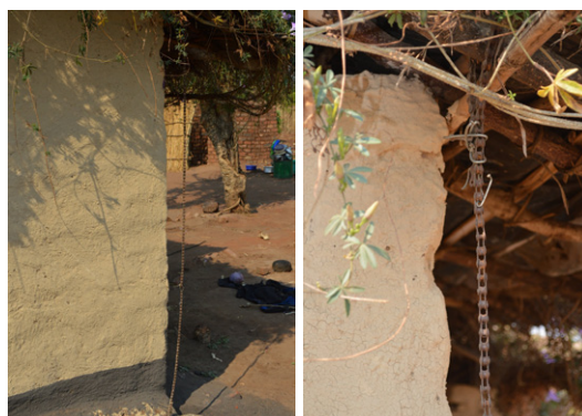
The roof structure is fastened to the ground with a motorcycle chain, what provides an additional connexion thus preventing the roof from being entirely blown off under wind pressure. House in Nsangu, Salima. © Jon Twingi
