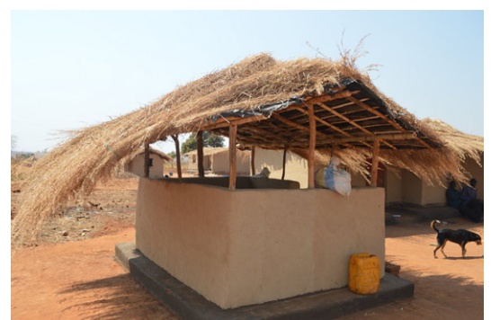
Kitchen with the upper parts of the walls open for improved ventilation. Nkhombe, Kasungu. © Jon Twingi
