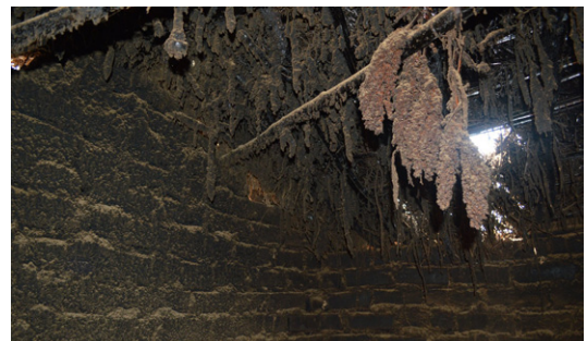
The use of CGI sheets without false ceilings and without ventilation in the gables causes thermal and acoustic discomfort. Market in Lilongwe. © Roderick Vd.
