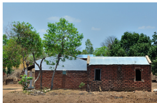
Corrugated galvanised steel or iron sheets are the most common metal roofing system in Malawi. Houses in Makala. CC- Hansueli Krapf
