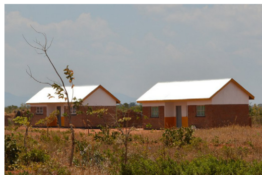
Houses with burnt brick walls, Reinforced Concrete beams and window sills, CGI sheets roof in Chisusu, Nzimba. © Jon Twingi
