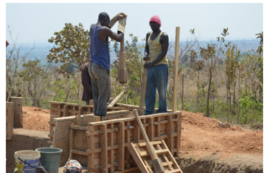
Many constructions in Malawi are built using local, renewable materials with little impact in the environment when they are well managed. This image shows the construction of a rammed earth house in Nisanje, Lilongwe. © Jon Twingi
