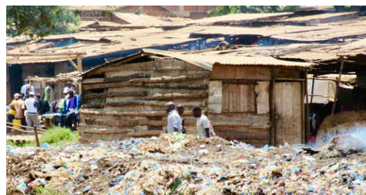
Precarious housing in Lilongwe. © Rethink Earth
