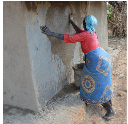
Women are involved in the construction, maintenance and protection of houses against particular hazards. Houses become more resilient thanks to this knowledge and know-how. Woman plastering in Chisi, Nzimba. © Jon Twingi
