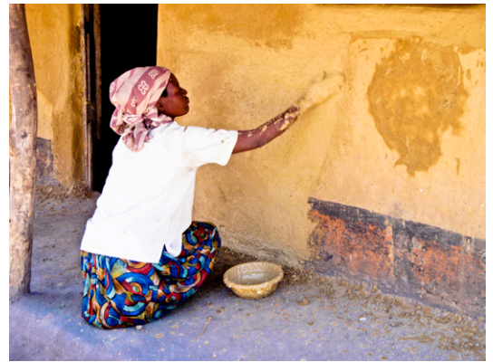
Woman cladding a wall with earth plaster. CC- Gregory S.
