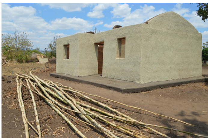
Rammed earth house under construction. © Jon Twingi
