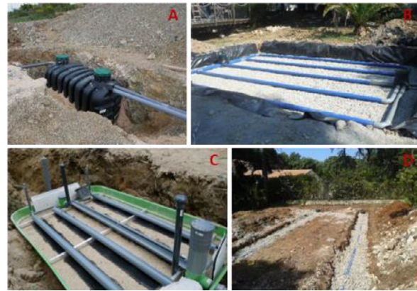
Fig. 1. Schematic representation of a septic system (adapted from EPA (2005)) and illustrative photos before filling operation (© KD, A: septic tank, B: sand filter, C: media filter, D: drain field).
