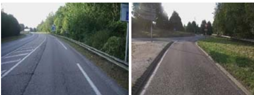
Fig. 5. Photographs of the marking line on Area 3. On the left, beginning of the line with presence of zebras; on the right, end of the line with presence of a pavement separator.
