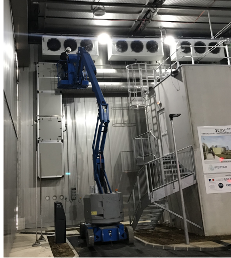
Figure 2: Partial view of the chamber ventilation system, including blocks of fans and a part of a set of suction and forced-air ducts. Picture taken during an experiment to measure the inflow velocities of the ventilation system of the climatic chamber using a 1D hot wire anemometer.
