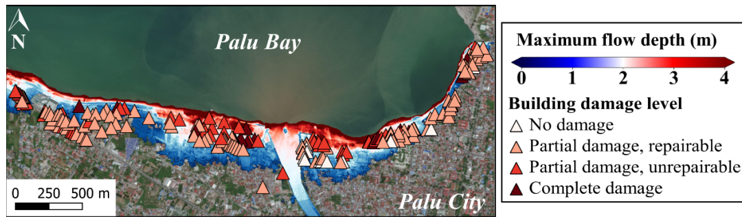
Figure 8. Sulawesi–Palu final tsunami inundation model with the maximum simulated flow depth overlaid on the damaged building data (background ESRI).
