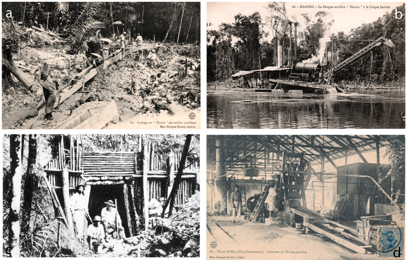
Fig. 5. Gold mining techniques used in French Guiana before WWII. a) Creole marauders working a sluice on an alluvial placer. Sluices are amongst the earliest artisanal methods used in French Guiana (postcard circa 1904; A. Heuret Collection); b) The Danica dredge, operated on the Sparwine River (Maroni region) since 1903, one of about twenty dredgers used along French Guiana rivers from the end of the 19th century. Dredges also marked the beginning of mechanized mining, which allowed gold to be extracted from untouched alluvial deposits in streams and swampy areas (postcard edited around 1904; A. Heuret Collection); c) Mine gallery entrance with wooden support structures. From the 1880s, this type of method was typically used for underground mining of quartz-bearing veins (picture taken in the late 19th century and edited for a 1930s postcard; A. Heuret Collection); d) Gold plant installed in 1898 at Adieu-Vat near Saint-Élie. The three-pestle Fraser & Chalmers crusher made it possible to extract gold from primary quartz ore. This plant marks the beginning of mechanized gold mining in French Guiana (postcard circa 1904; A. Heuret Collection).
