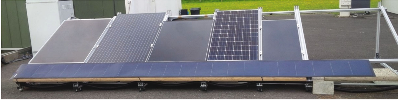
FIGURE 2: Outdoor characterization PV platform located at SIRTa.
