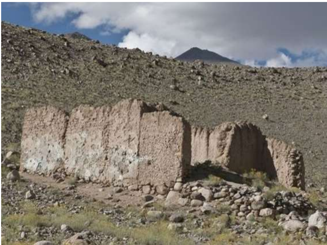
Fig.9: general view of the main temple (Co1) of Leh Choskor looking north-west.
