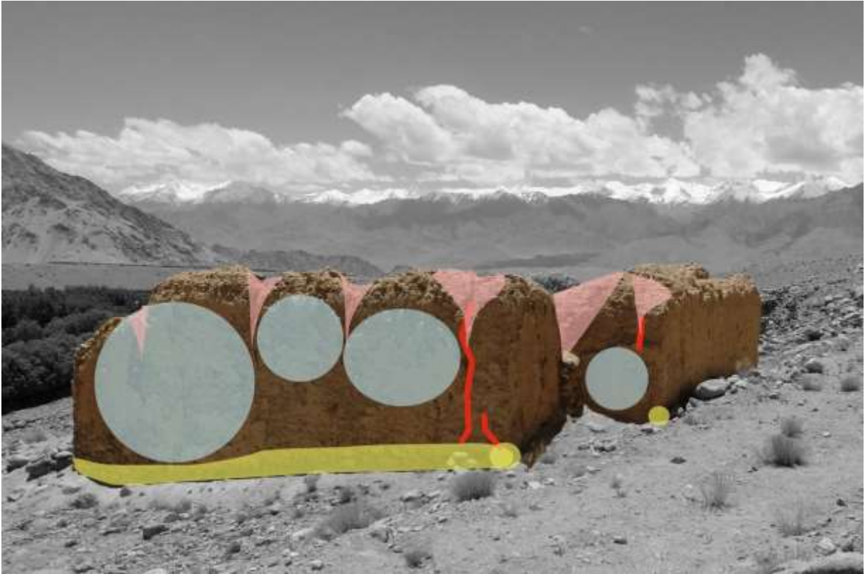
Fig. 22: pathologies on the outer side of the northern wall, temple Co1, Leh Choskor. ©MAFIL/Sadozai.
