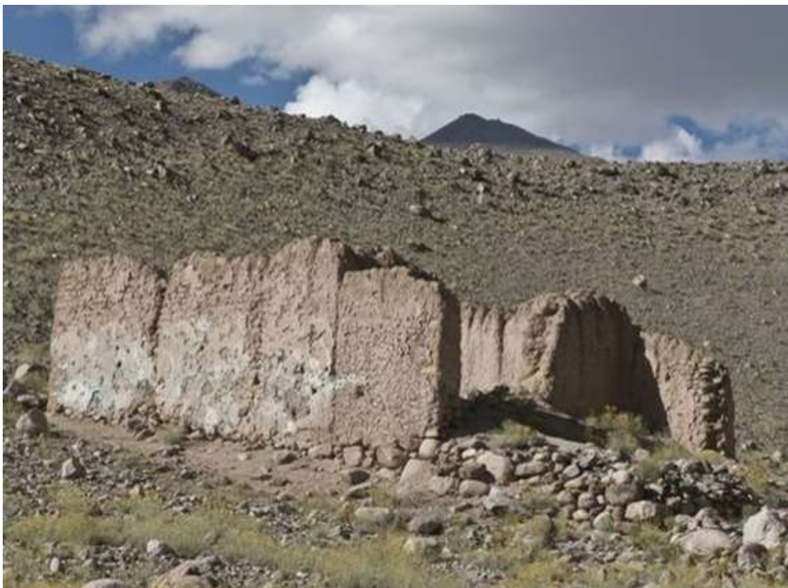
Fig.9: general view of the main temple (Co1) of Leh Choskor looking north-west.
