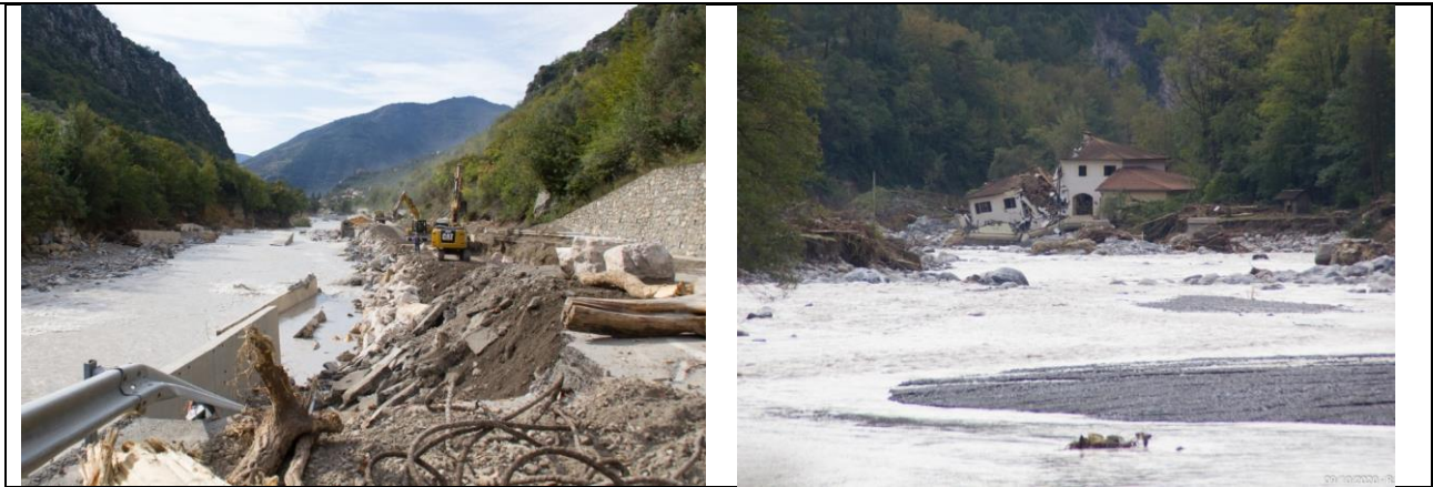
Figure 11: Road access to the south of Breil-sur-Roya are destroyed, while a temporary unpaved road is being created (left picture). A house has been cut in half by the Roya floods (right picture).
