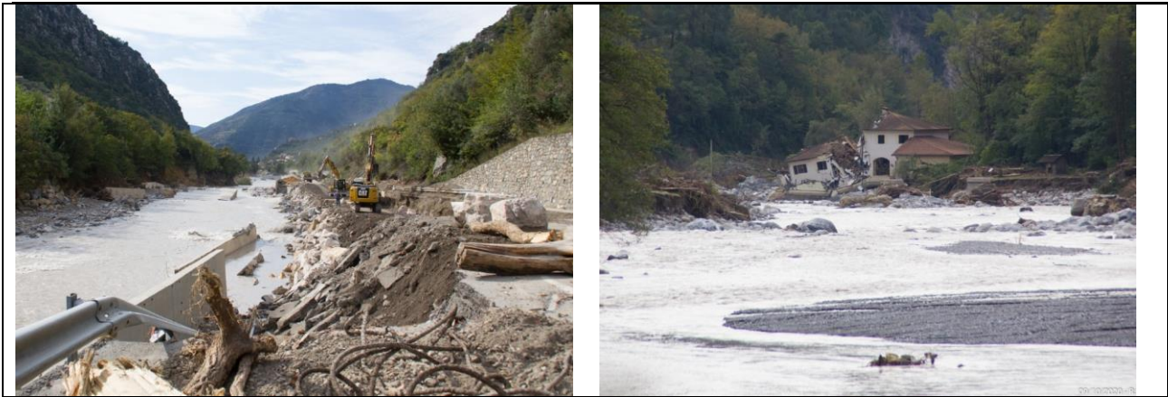
Figure 11: Road access to the south of Breil-sur-Roya are destroyed, while a temporary unpaved road is being created (left picture). A house has been cut in half by the Roya floods (right picture).
