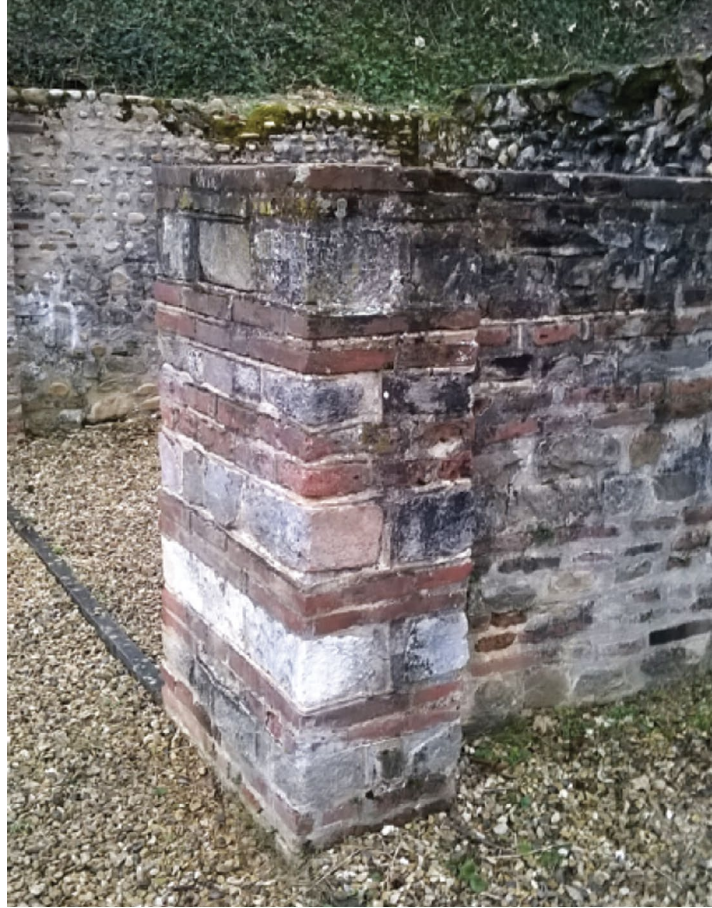
Fig. 7: Pillars in mixed opus of the shops at the back of the odeon.
