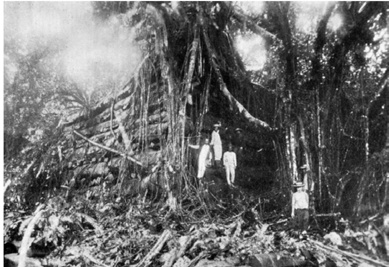
Figure 5. View of the north-east corner of Nandowas taken in 1896, showing the large banyan trees topping the walls (in Christian 1899a, p. 102a).
