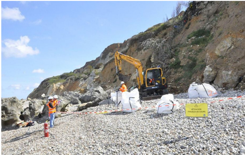
FIGURE 6 | Trial waste removal at the Dollemard landfill (summer 2020). Photograph courtesy of Le Havre council.
