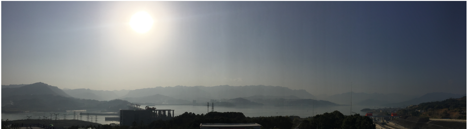
Figure 12. The Three Gorges Dam and the reservoir, Yichang (Hubei) China. Source: Katiana Le Mentec, 2017.
