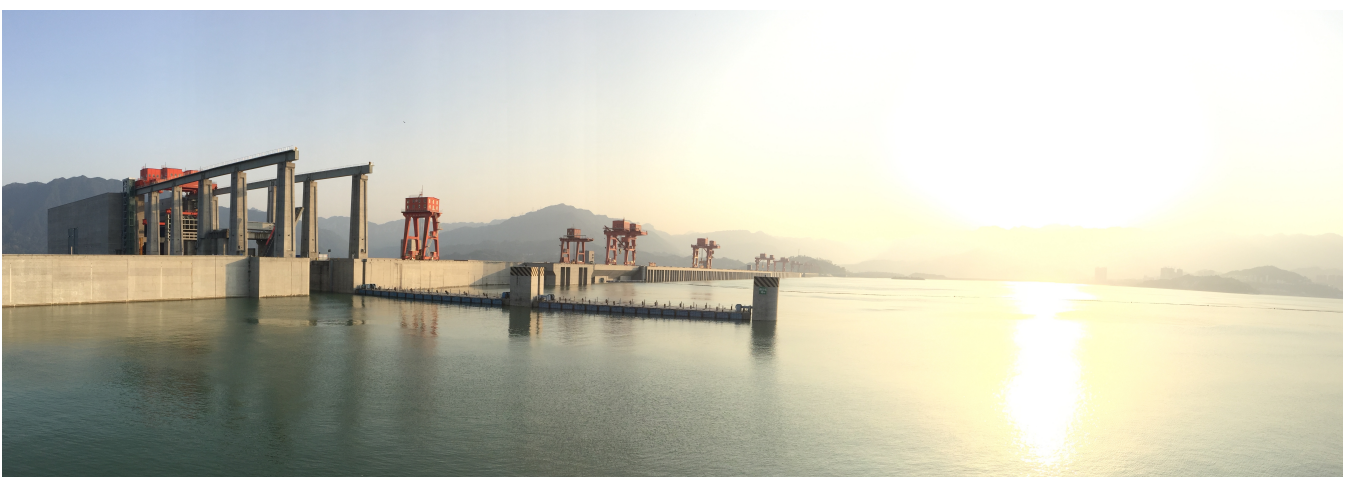
Figure 3. The Three Gorges Dam from the Three Gorges Reservoir, Yichang (Hubei) China. Source: Katiana Le Mentec, 2017.
