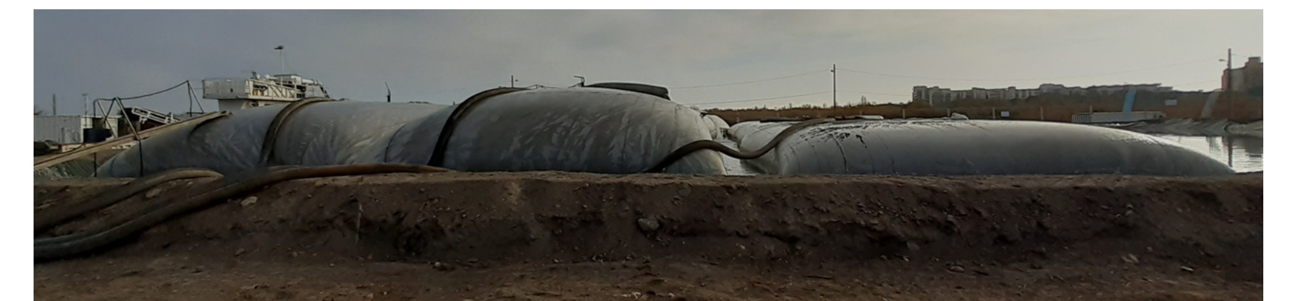
Drainage in geotubes - Pérols (Sordes 2020)
