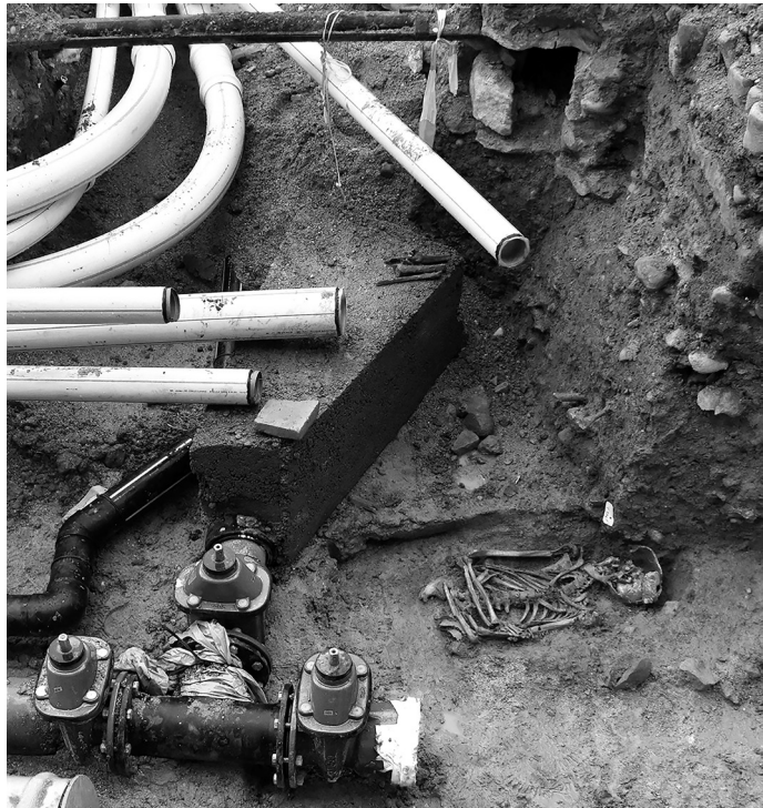
Figure 9. Grandson view of trench excavation (Archeotech SA).
