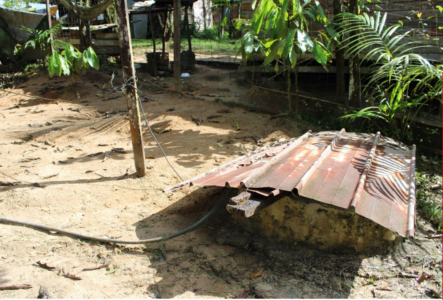
Fig. 4 : well n°3, a type of "Amazonian" (dug) well, covered with cleats
