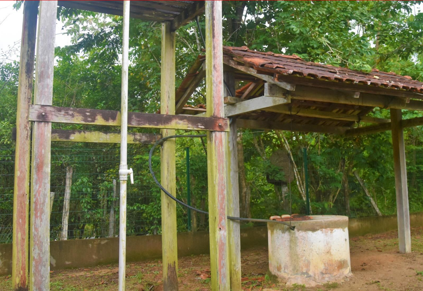
Fig. 3 : well n°4, a type of "Amazonian" well (dug), covered with cement and roof
