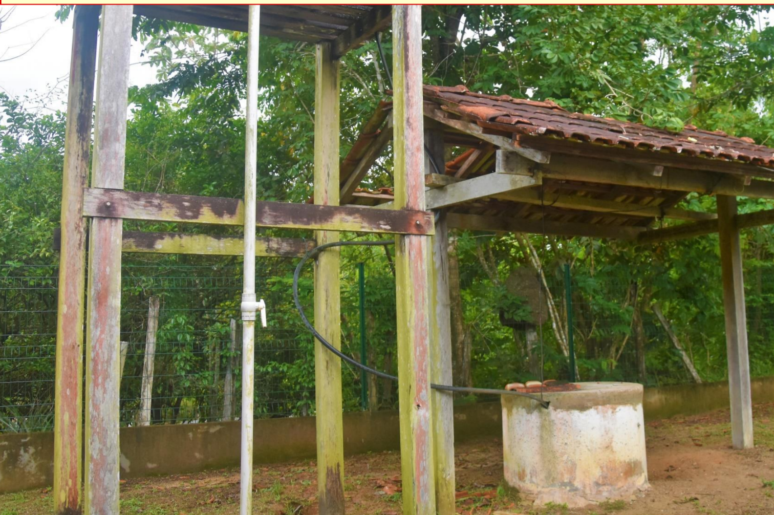
Fig. 3 : well n°4, a type of "Amazonian" well (dug), covered with cement and roof
