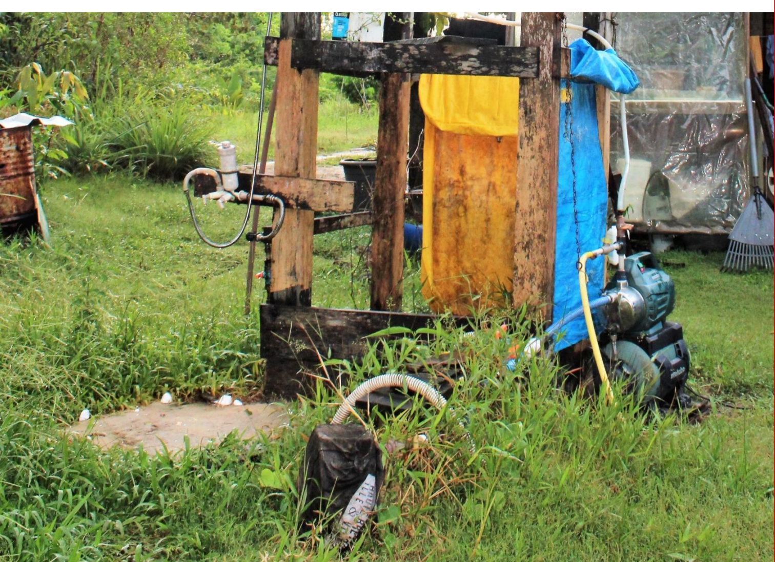
Fig. 5 : well n°8, a type of "artesian" well (drilled) with an individual filter
