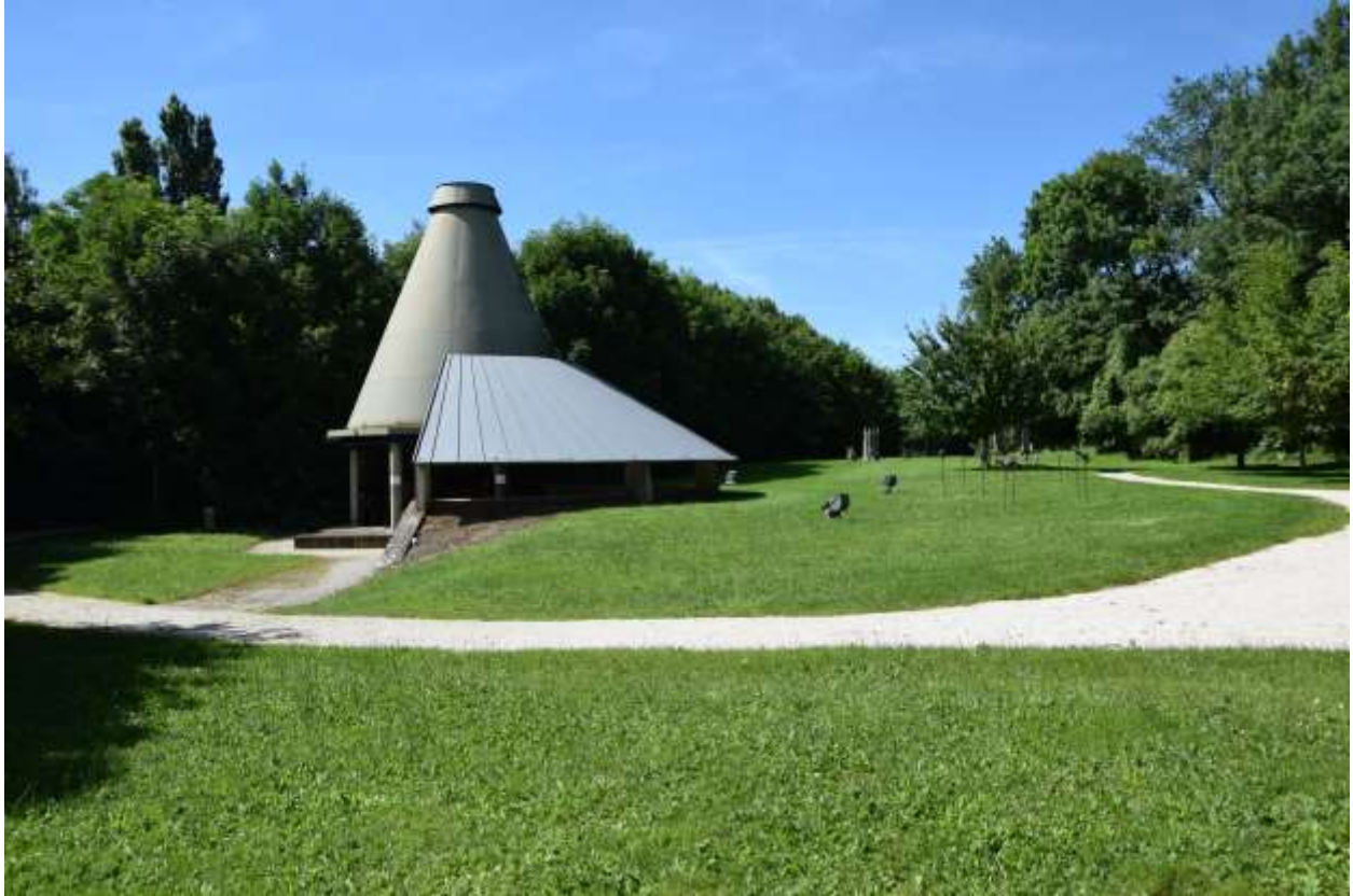
Figure 1: The central structure at Melle, within which a large forge and closed ovens are housed (left) and visitors to the experimental platform (right).
