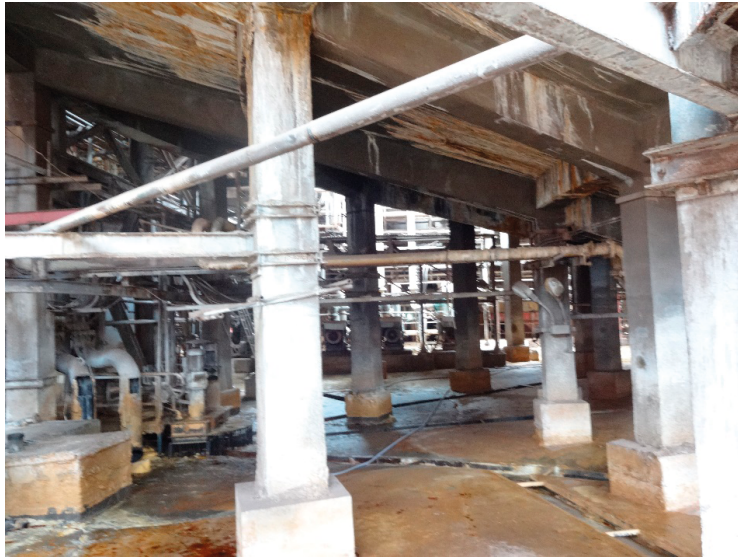
Figure 1. A RCC tertiary thickener structure of Alumina plant rests on concentric columns
