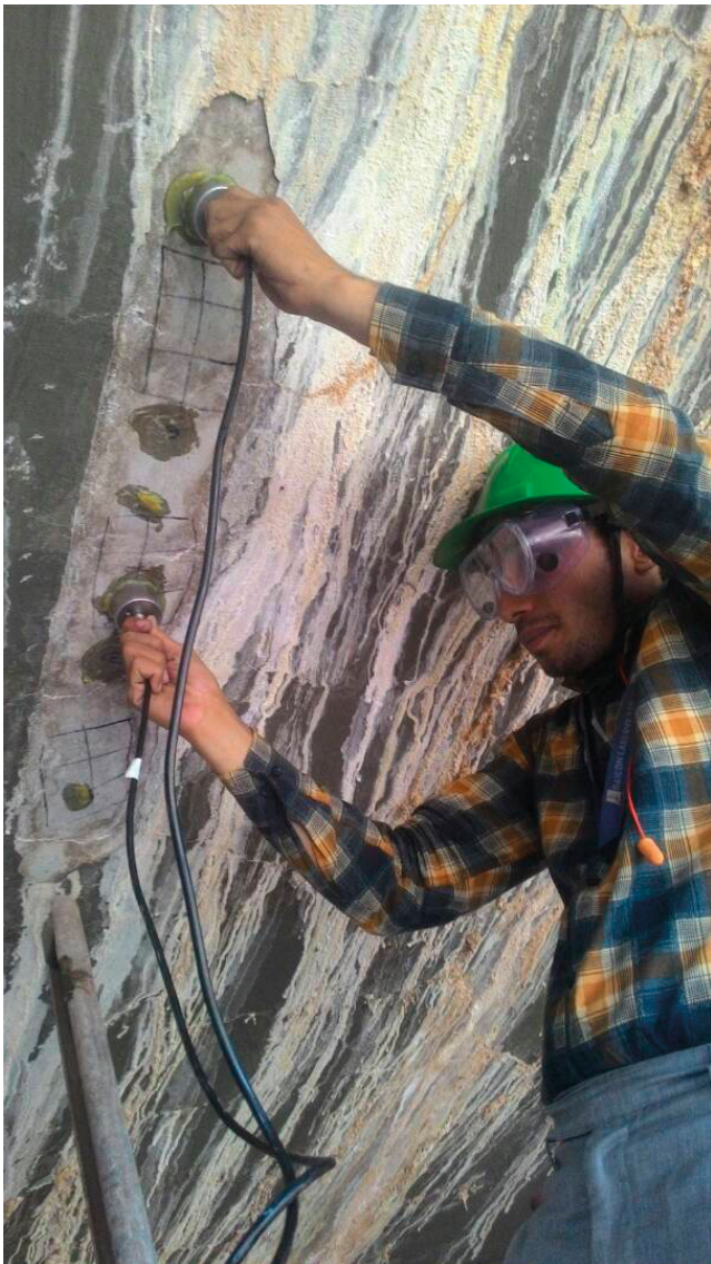
Figure 2. Ultrasonic pulse velocity test
