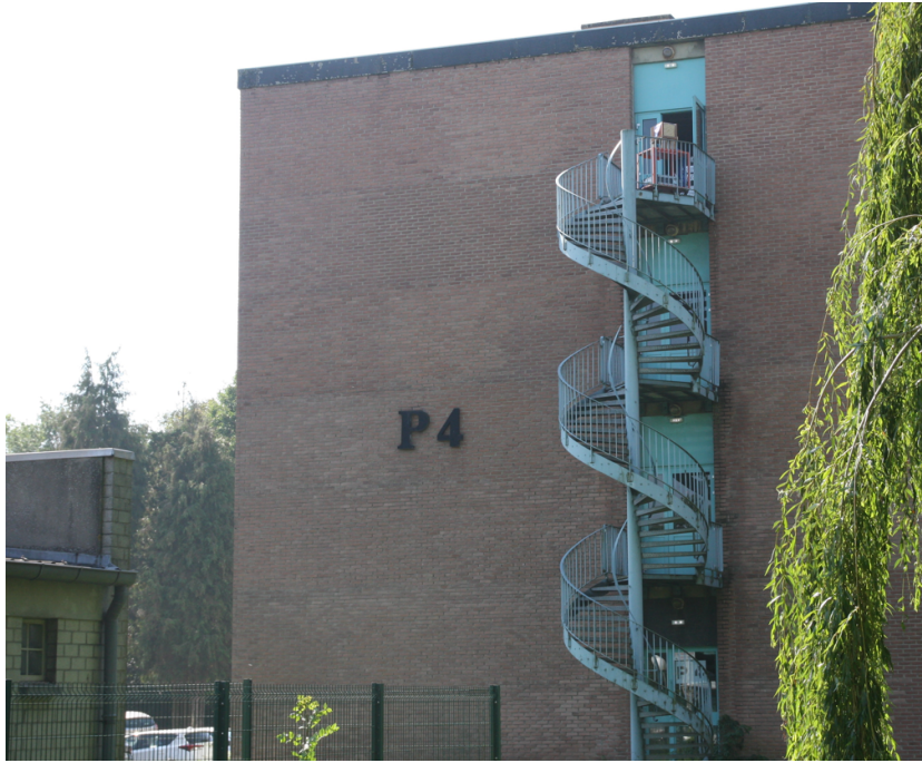
Figure 2. Tx on the P4 building platform
