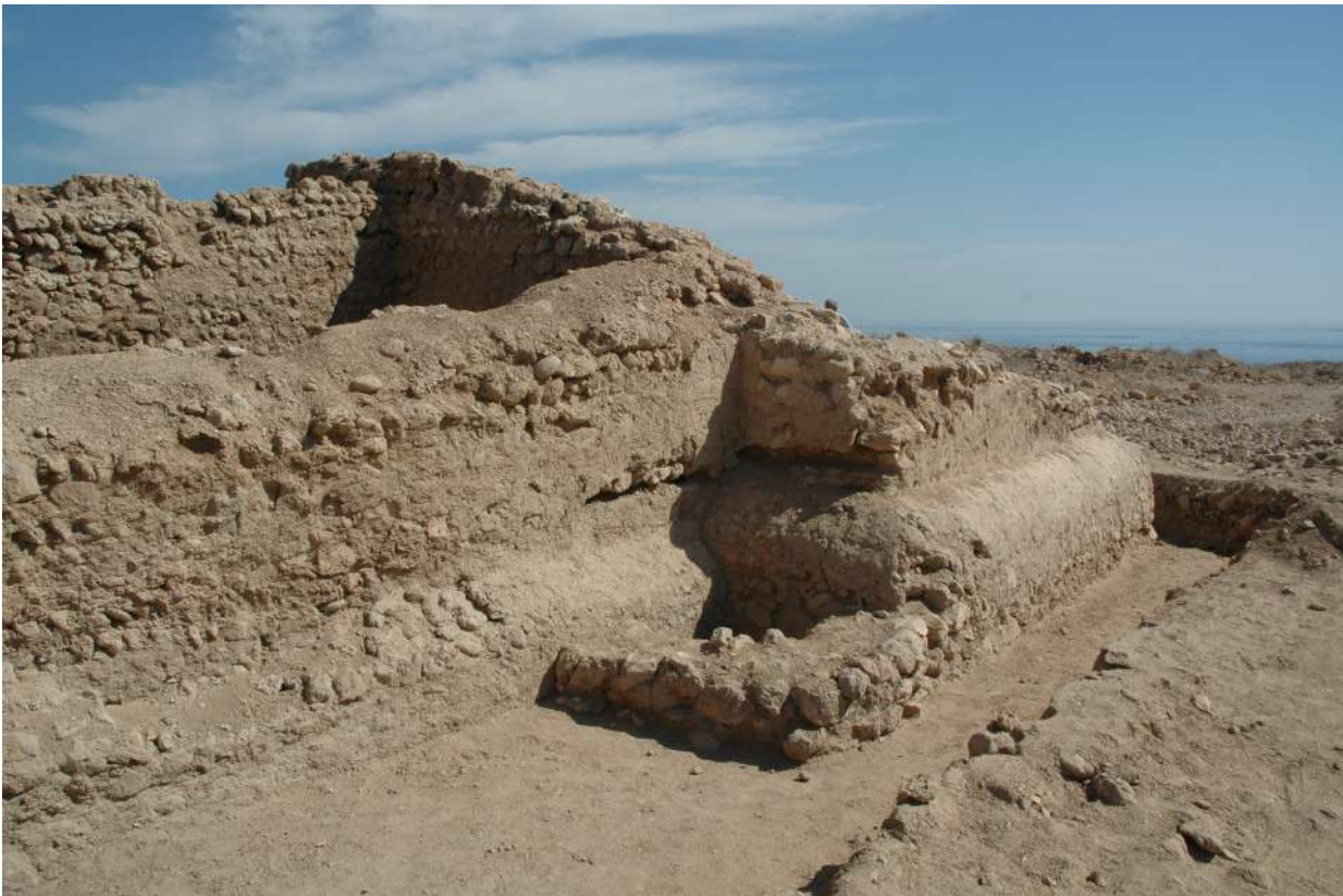
Fig.43_The buttress around the south-east corner of the house
