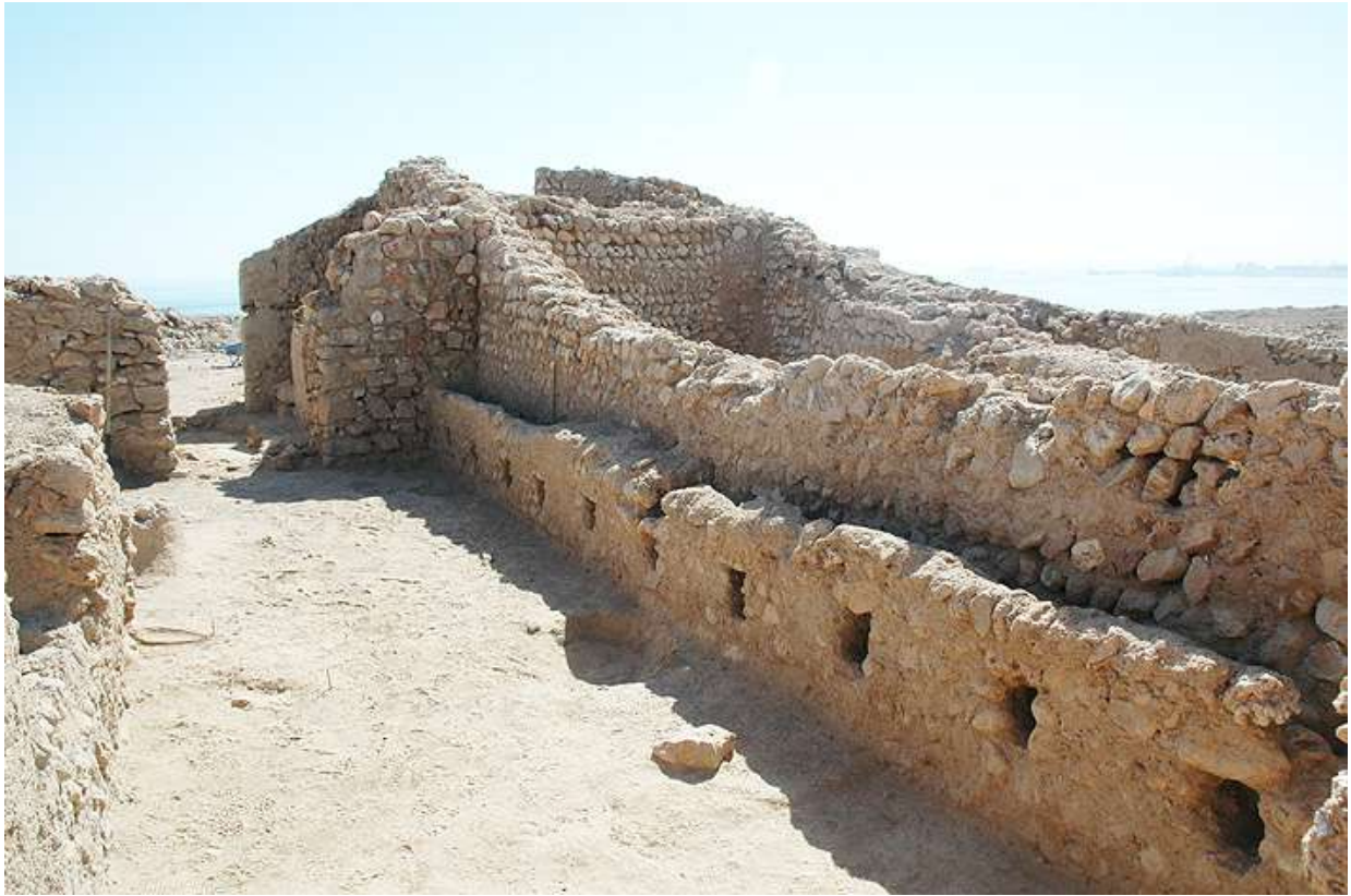
Fig.22_structure ST 050 along the southern wall of the courtyard B94D
