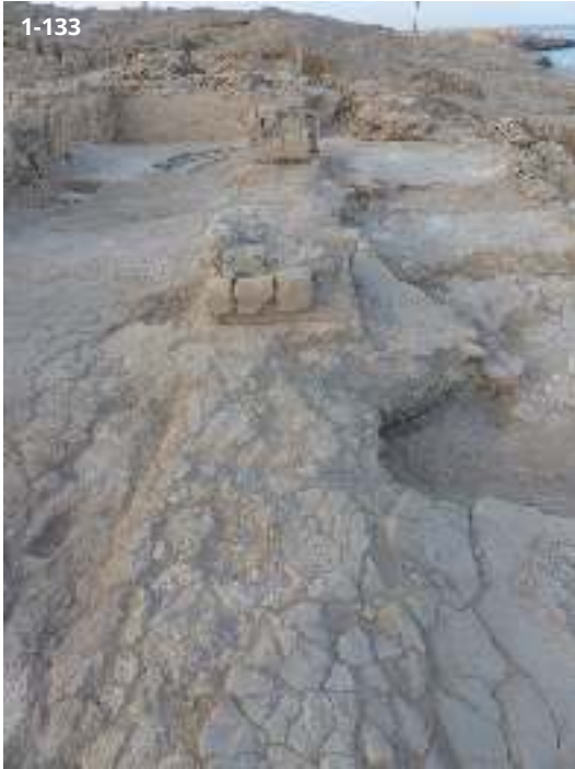
Fig 1-133 : the intermediary wall B12-45 under the row of pillars, visible by the cracks of the floors, in the south part
