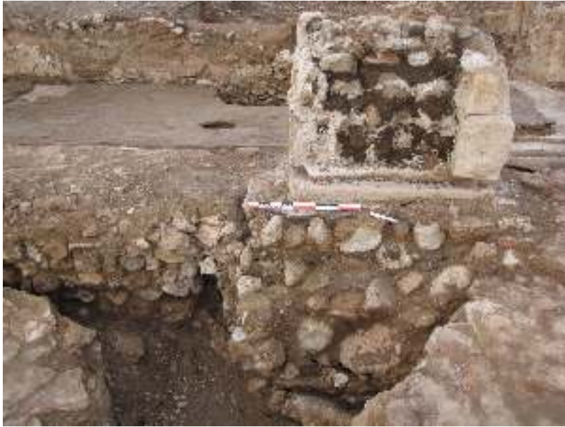
Fig 1-165 : the reinforcement B12-356 under the pillar B12-232
