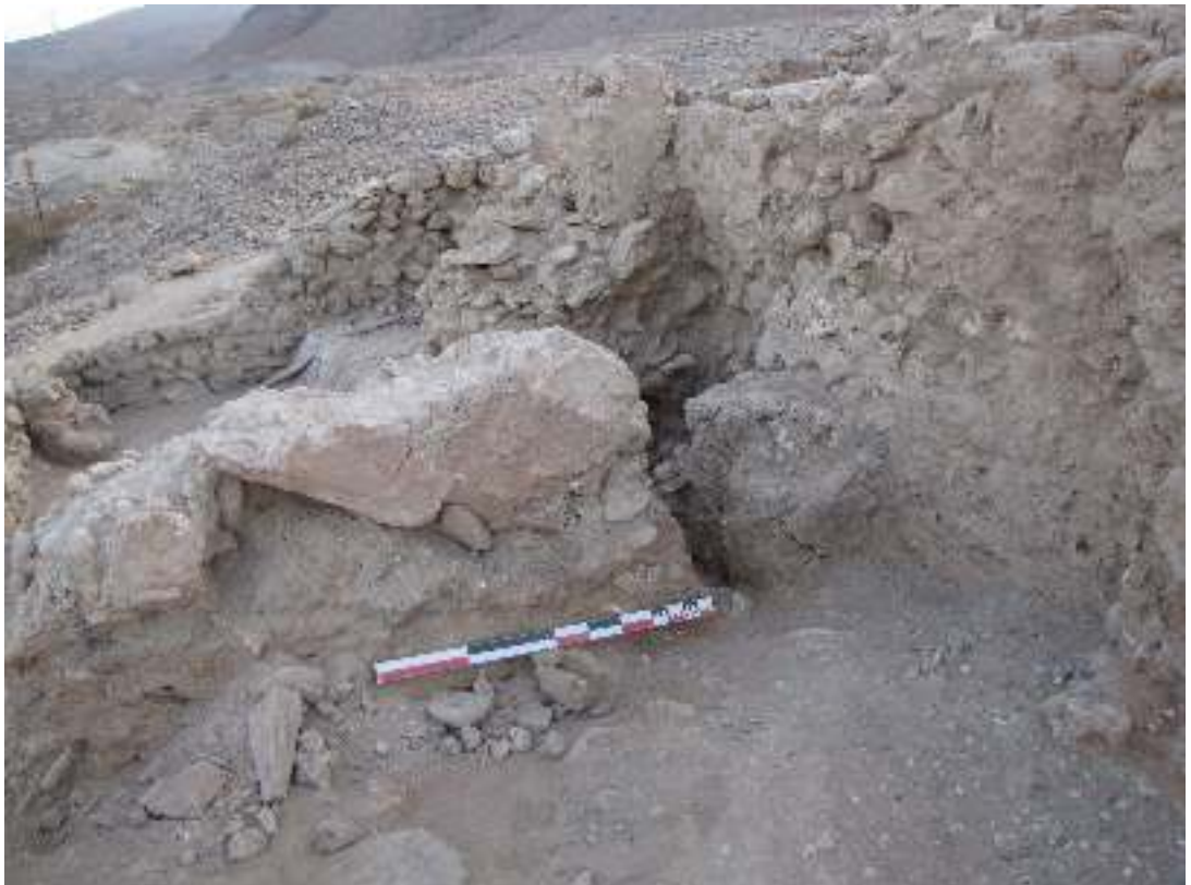
Fig 1-8 : the buttress B12-347, at right of the fallen pillar that was once standing above
