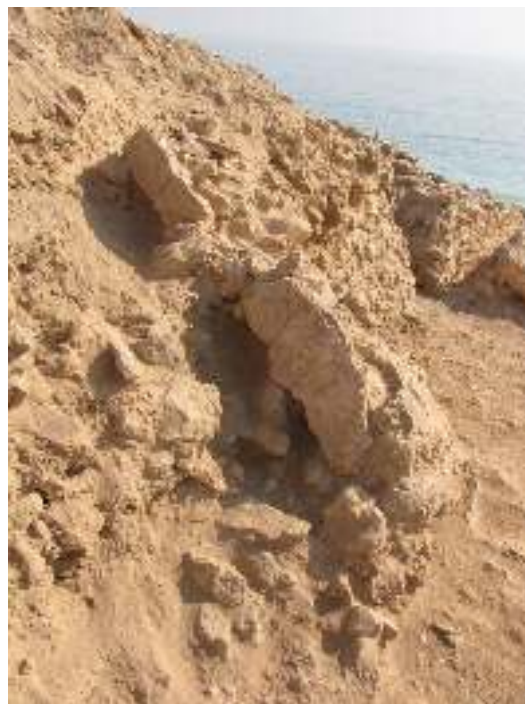
Fig 1-280 : imprints in the mortar of the wall B12-41, suggesting the presence of a disappeared buttress
