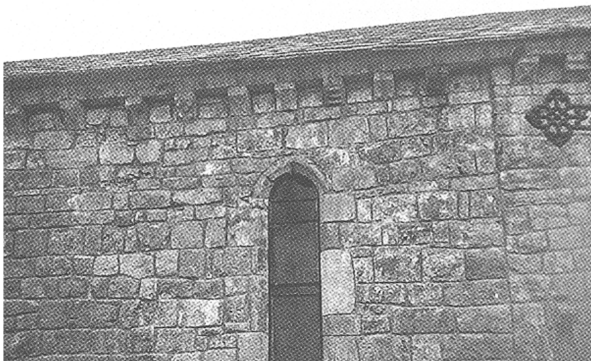
Figure 4. — Lanuéjols. Façade sud, chapelle.
