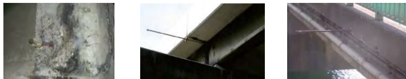
Fig. 1 Rupture and protrusion of PC bar tendon [9], [10], [14]
