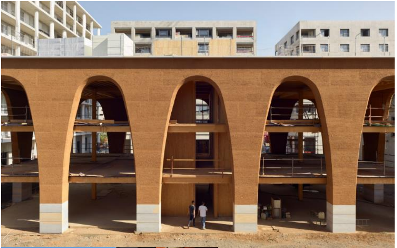
Figure 1: the “Orangerie” rammed earth building during its construction in the centre of Lyon (top, © Fabrice Fouillet). The arches are load-bearing structure holding the timber floor and the flat roof. The timber floors are ensuring safety against earthquakes by tying the facades together and connecting them to the vertical timber structure around the lift (in the middle, of the photo). The partial on-site automation of the construction enabled to deliver the project with reasonable cost and time. Down left: A single-family house in rammed earth, Burgundy, France (© Nicolas Meunier).
