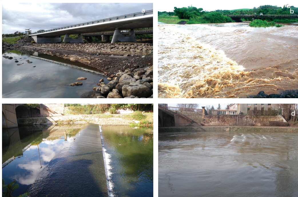
Examples of structures under different discharge conditions. Glacis on the Sainte-Suzanne River on Réunion under low-flow (a) and high-flow (b) conditions. A weir in continental France under low-flow (c) and high-flow (d) conditions.
