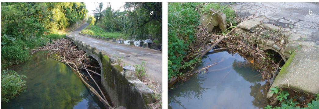
Examples of structures significantly blocked by debris. (a) and (b) Blocked structures on rivers on Martinique.
