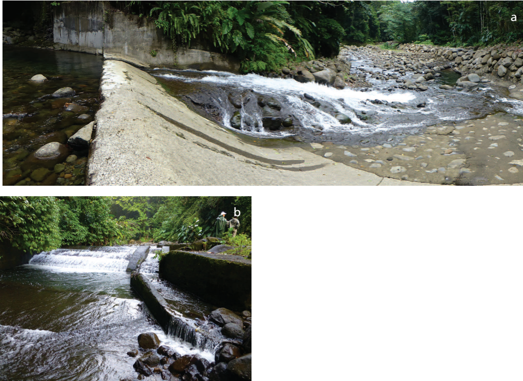
Examples of complex structures that can be broken down into a series of "simple" structures. (a) A structure that can be broken down into an inclined weir and a downstream rock weir (Pérou River, Guadeloupe), (b) A structure that can be broken down into two successive inclined weirs (Saint-Louis River, Guadeloupe).
