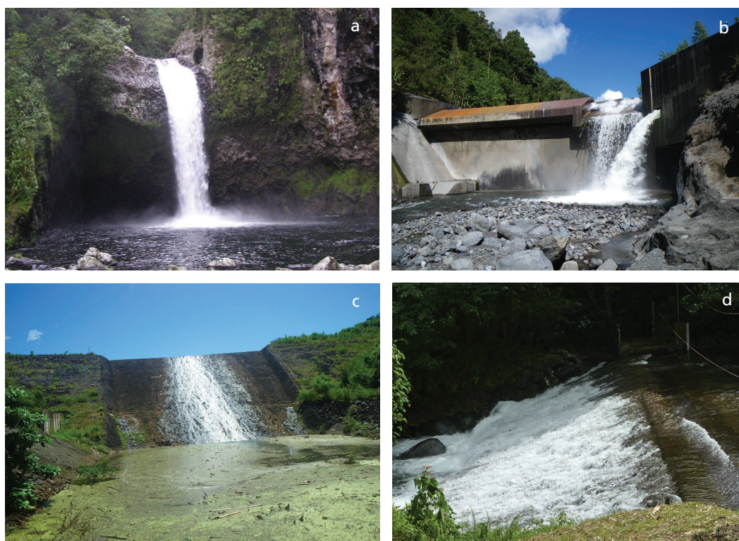
Examples of spillways and natural waterfalls that fish must overcome when migrating downstream. (a) Natural waterfall (Réunion), (b) Vertical waterfall over a dam spillway (Réunion), (c) Water flowing over the glacis of a dam (Mayotte), (d) Water flowing over a glacis (Martinique).
