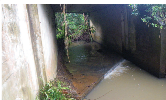
Example of very low water depths on the apron of a road bridge. Passage of the Beja River (Mayotte).
