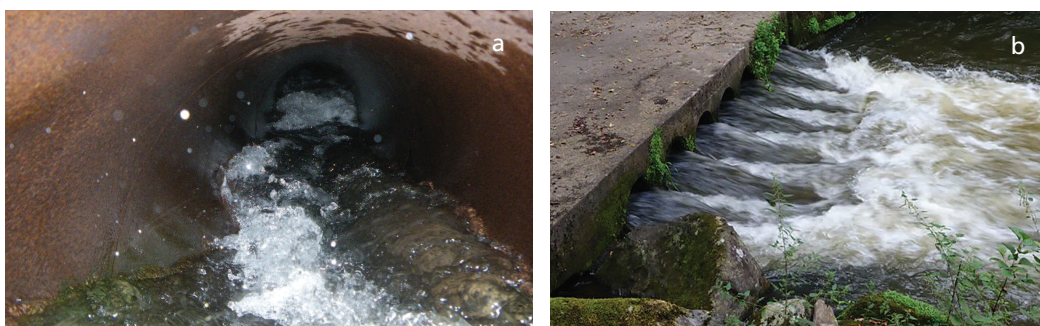
Examples of high flow velocities in culverts. (a) Culvert on the Saint-Étienne River (Réunion), (b) Ford over the Maronne River (continental France).
