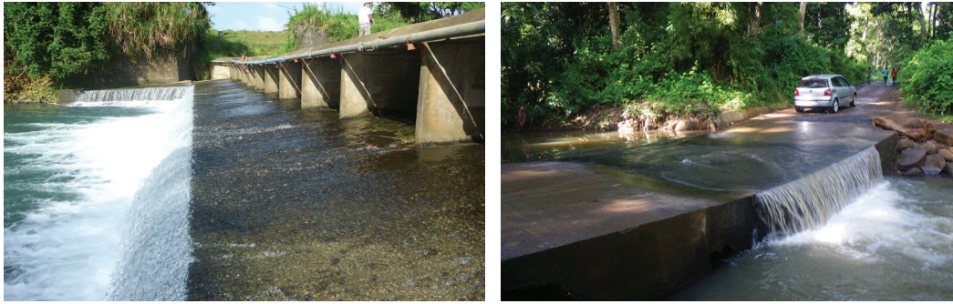
Flow over an inclined downstream face with a downstream waterfall. (a) Goyaves Grande River (Guadeloupe), (b) Moala ford on the Orouvéni River (Mayotte).
