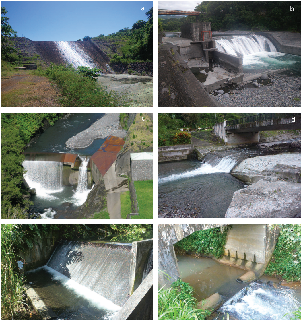
Examples of weirs and dams on rivers in the French insular, overseas territories. (a) Dzoumogné reservoir for drinking water (Mayotte), (b) Bengalis weir for irrigation on the Mât River (Réunion), (c) ILO weir for irrigation on the Mât River (Réunion), (d) Stabilisation weir on the Grande River (Martinique), (e) EDF weir (drawoff for hydropower) on the Bananier River (Guadeloupe), (f) Hydrometric weir (Martinique).
