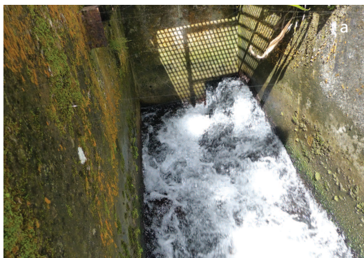
Example of a structure that cannot be broken down into "simple" structures. In this case (controlling flow under a gate, followed by an inclined weir), the structure cannot be broken down into two "simple" structures. Due to the gate configuration, the initial velocity at the head of the inclined face is much higher than for a normal inclined weir on which the velocity increases progressively. Note that hydraulic modelling would be of no use in this case because passage under the gate is not possible. The overall structure may be considered a total barrier (ICE class = 0).
