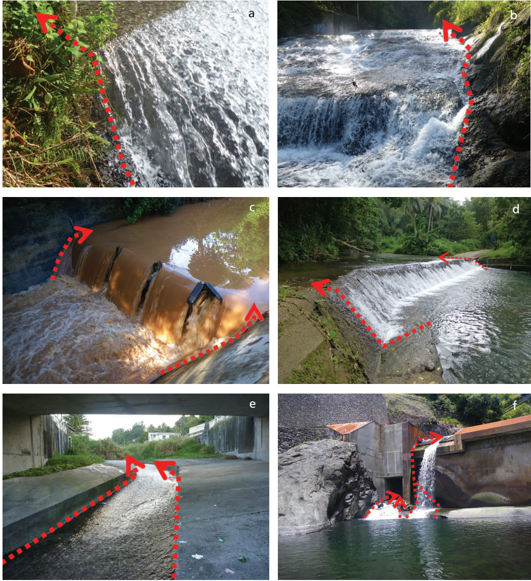
Examples of potential crawl ways for eels that should be analysed (marked by the red arrows). The arrows also represent potential passageways for Sicydiinae or the post-larvae and juveniles of small, benthic species using suction techniques and as walkways for macro-crustaceans (photos from Martinique, Mayotte and Réunion).
