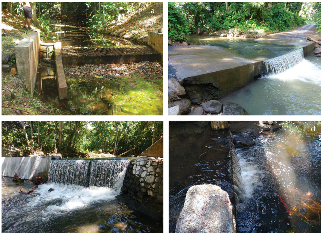
Examples of plunge pools at the foot of obstacles. (a) Insufficient pool, (b) Sufficient pool, (c) Insufficient pool, (d) Sufficient pool.
