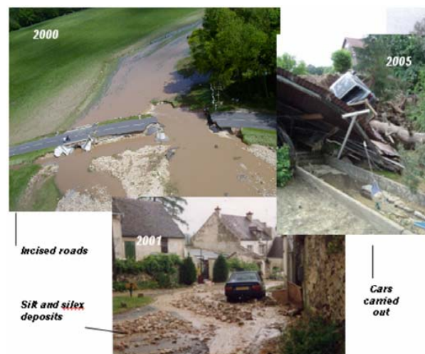
Fig. 1. Photographs showing the violence and impacts of flash floods occurring in the North of France during summer of at the end of the summer after high rainfall intensities (Douvinet, 2008).
