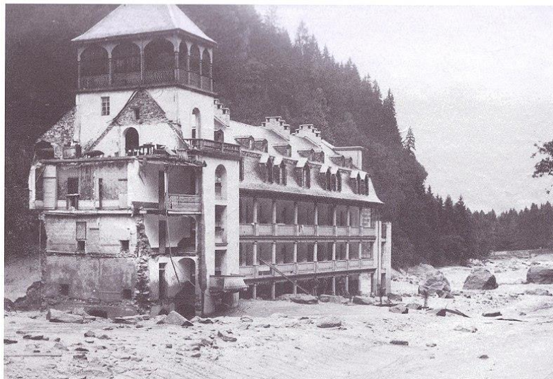
568 Figure A1. The wiped-out thermal bath of Saint-Gervais after the debris flow of the 12th of July 1892 569 (Thermes de Saint-Gervais Mont-Blanc, 2021).
