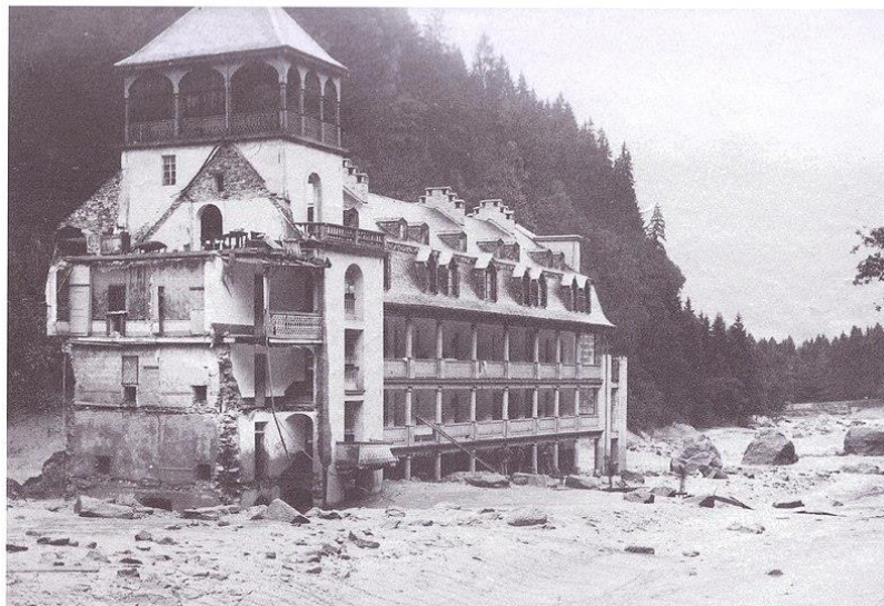
568 Figure A1. The wiped-out thermal bath of Saint-Gervais after the debris flow of the 12th of July 1892 569 (Thermes de Saint-Gervais Mont-Blanc, 2021).
