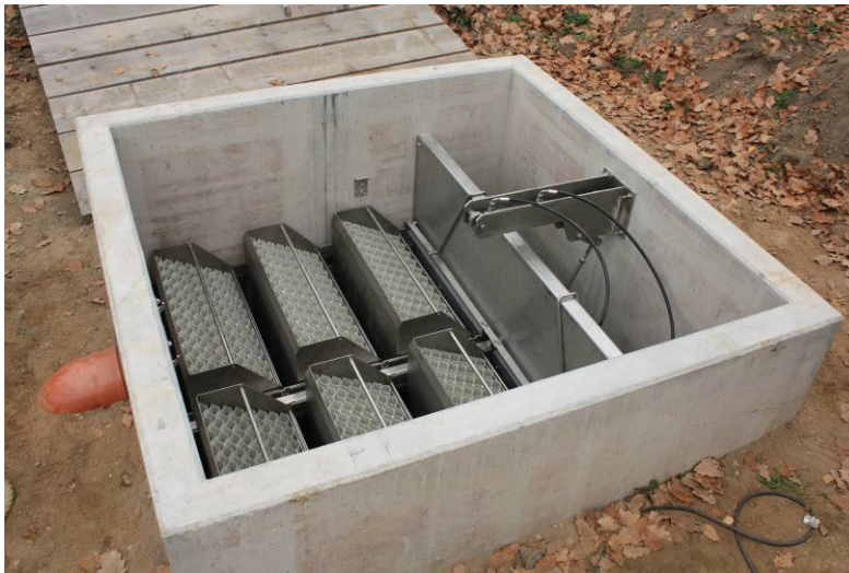
Fig. 8: For cleaning, the lamella modules are pivoting under water by a hydraulic drive. The sludge slides down and is drained to a sanitary sewer.
