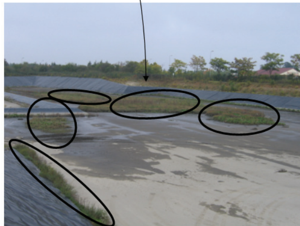
Figure 7 : Comparison between simulated - with the turbulent kinetic energy values below to 0.00002\text{ m}^2/\text{s}^2 and observed settling areas – Q_{\text{inlet}} = 1\text{ m}^3/\text{s}
