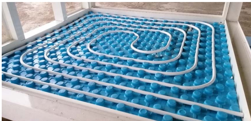
Figure 8 Hydronic pipes configuration at the prototype's floor.
