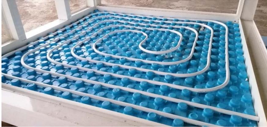
**Figure 8** Hydronic pipes configuration at the prototype's floor.
