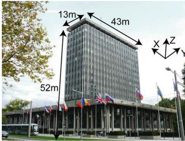
Fig. 1 CGH: view of the tower and the peripheral building
