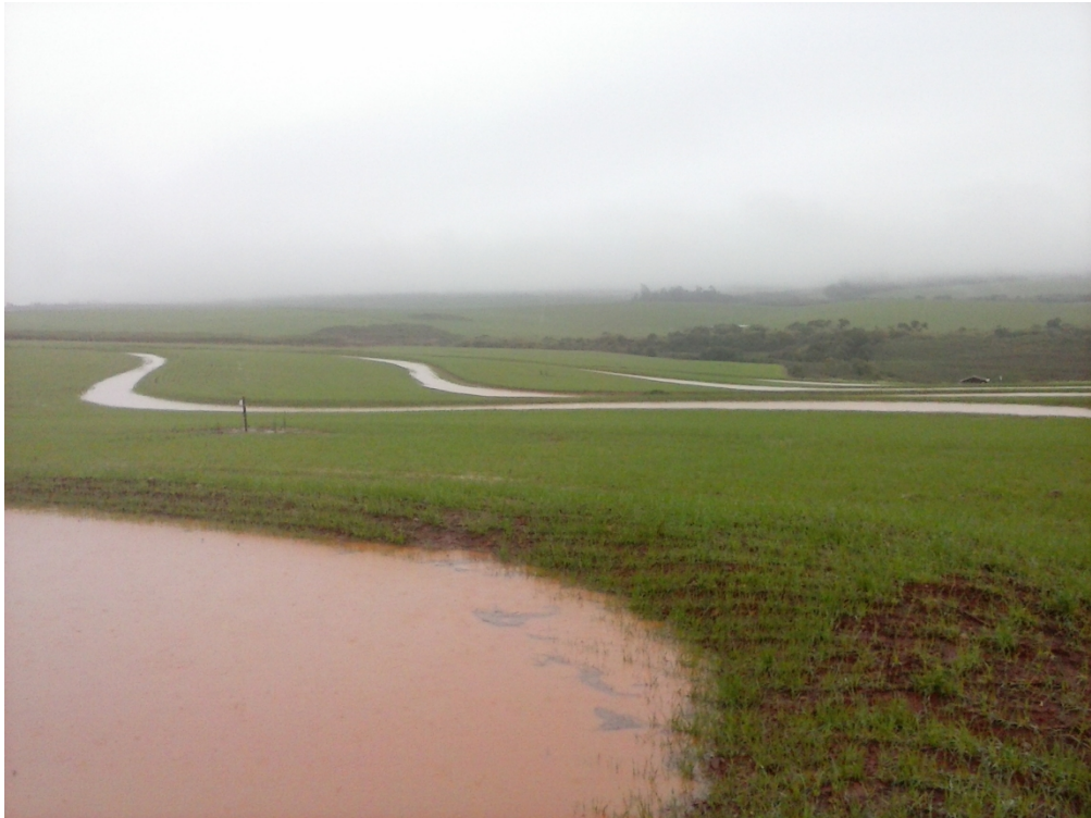
Figure 2. The terraces controlling the runoff after a rainfall event.
