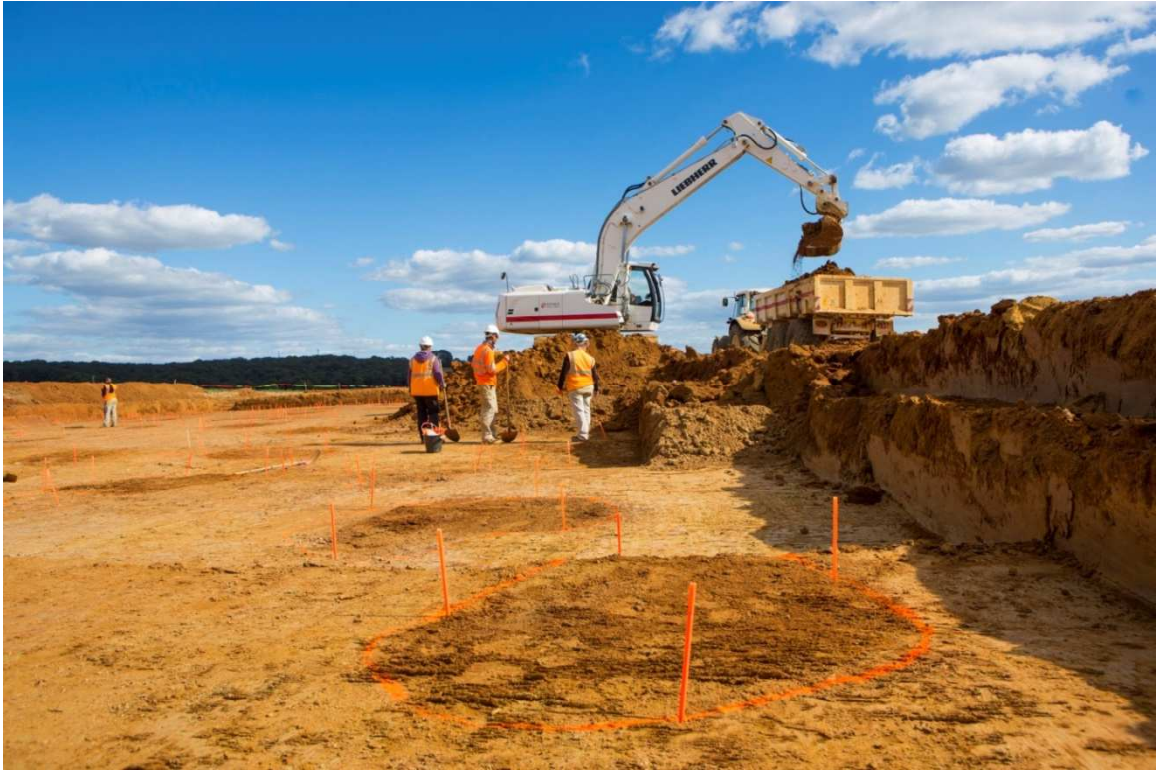
Figure 1 BPL high-speed line during construction [EIFFAGE rail express]
