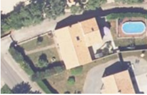
Figure 8: The detection of a window on a roof is immediate from the IGN cartography (47.183722, -1.812768) - © IGN 2018.
