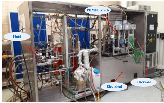
Fig. 1. The 10 kW experimental platform of the PEMFC system.
