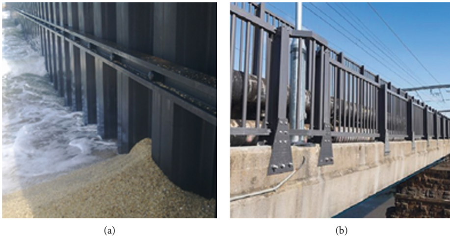
FIGURE 4: Pultruded retaining wall in Azerbaijan (a) and pultruded railway bridge barriers in England (b) [9, 10].
